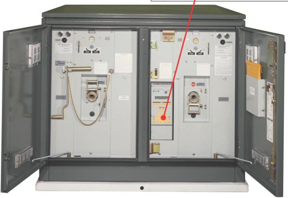
Figure 1. Micro-AT control installed in the S&C Source-Transfer Pad-Mounted Gear.
