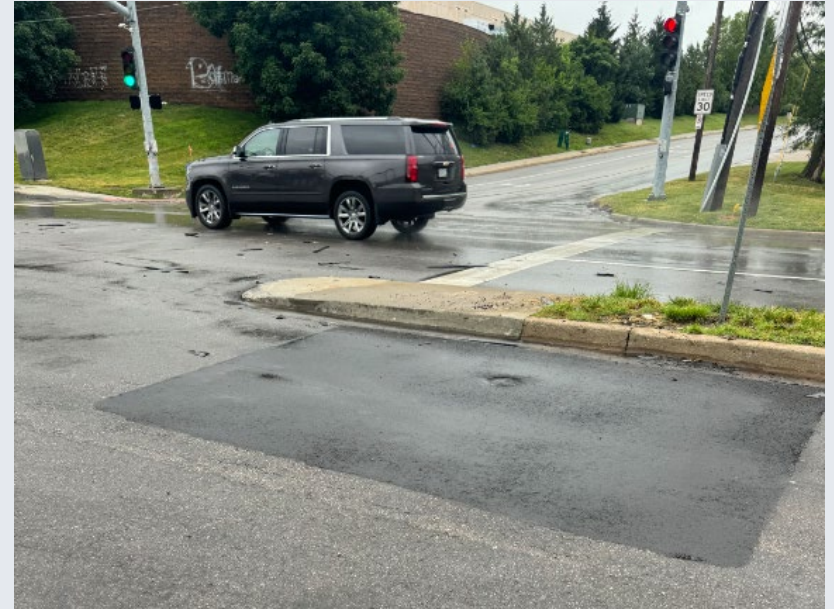
Restoration after valve replacement
