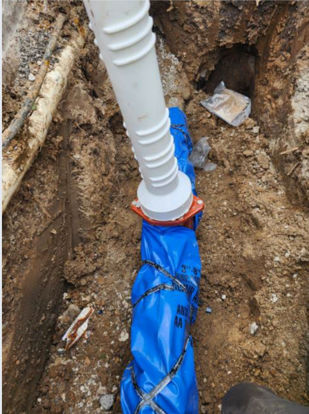
Replacement of an old water valve
