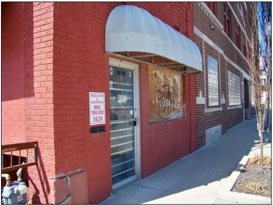
3634 Main St – looking northwest – deterioration of window
