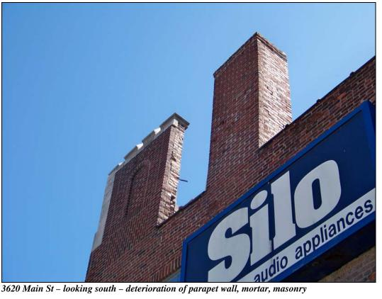
3620 Main St – looking south – deterioration of parapet wall, mortar, masonry
