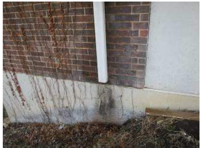
Poor Drainage &amp; Erosion – 2644
