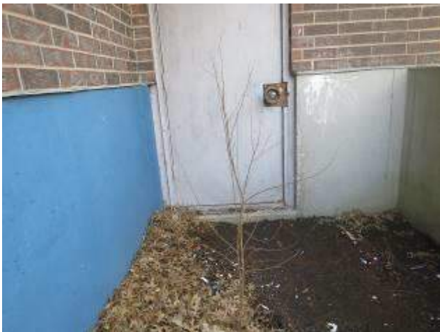
Poor Drainage At Entrance – 2644
