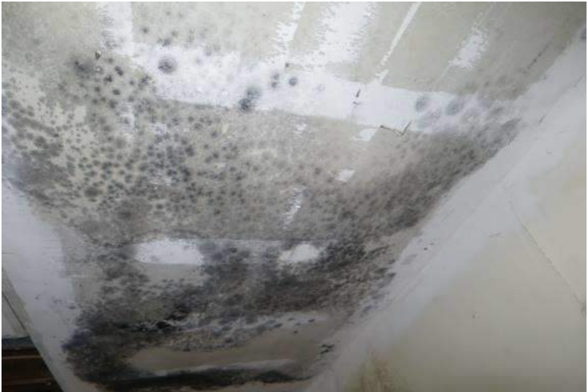
Water Infiltration & Potential Mold – 2644 E 29 th Street
