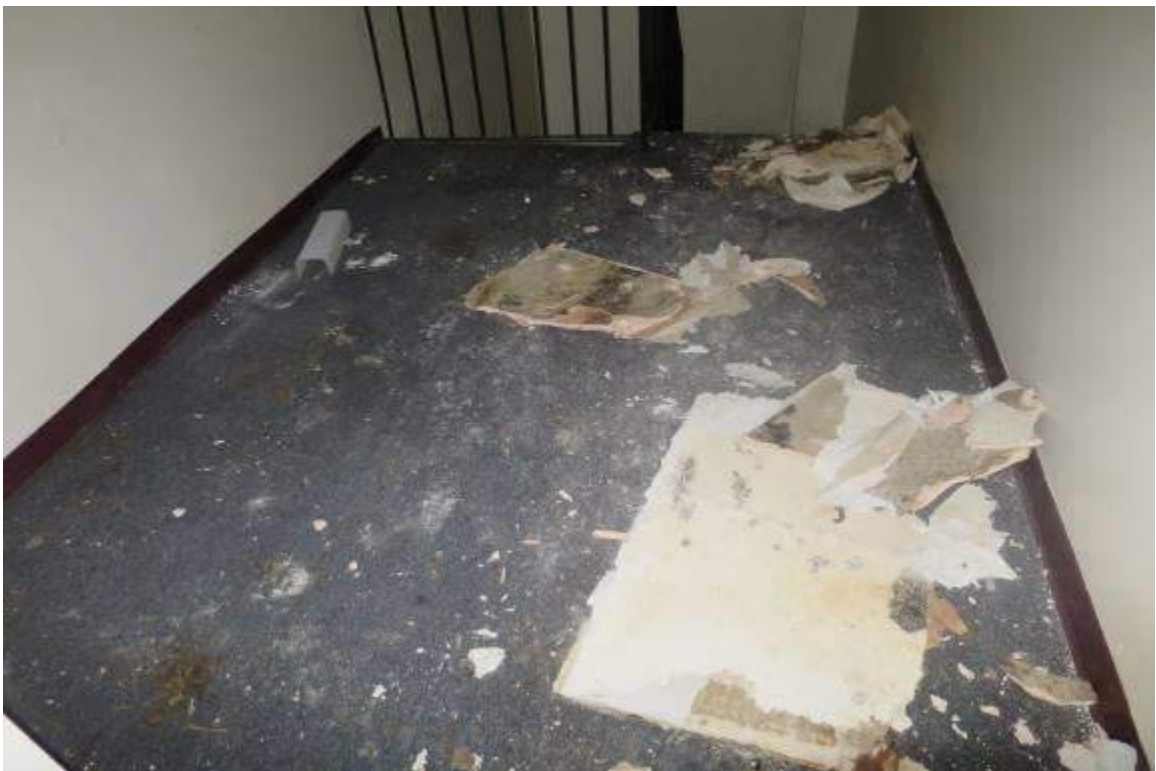
Collapsing Ceiling Structures – 2644 E 29 th Street
