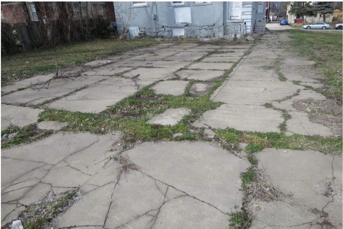
Damaged & Deteriorating Concrete-Paved Parking Area – 2651 Victor Street
