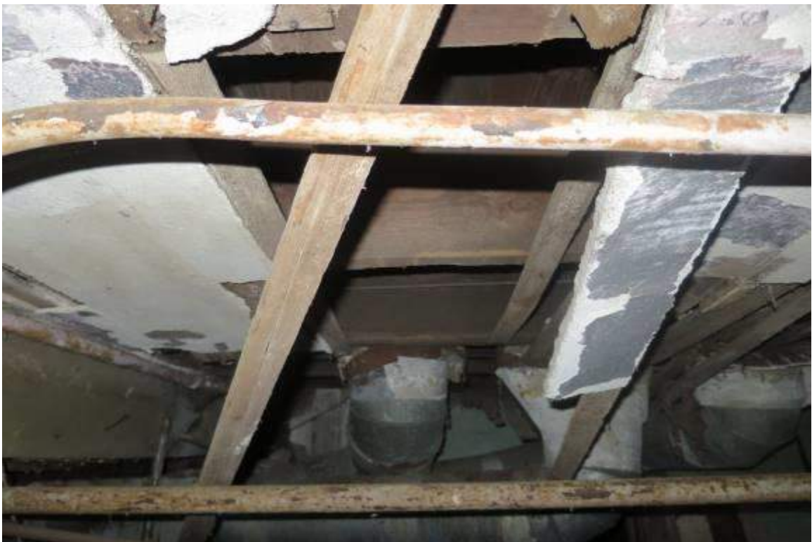
Potential Lead-Based Piping – 2651 Victor Street
