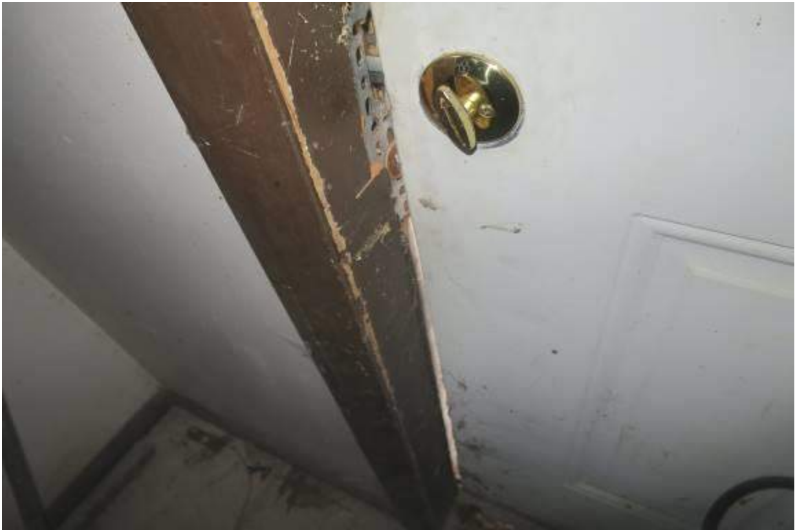
Damaged & Ill-Fitting Entry Door
