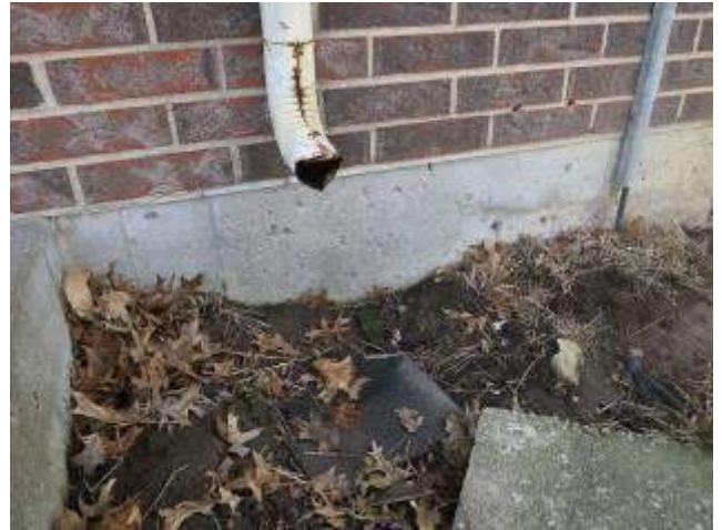
Poor Drainage &amp; Erosion – 2644
