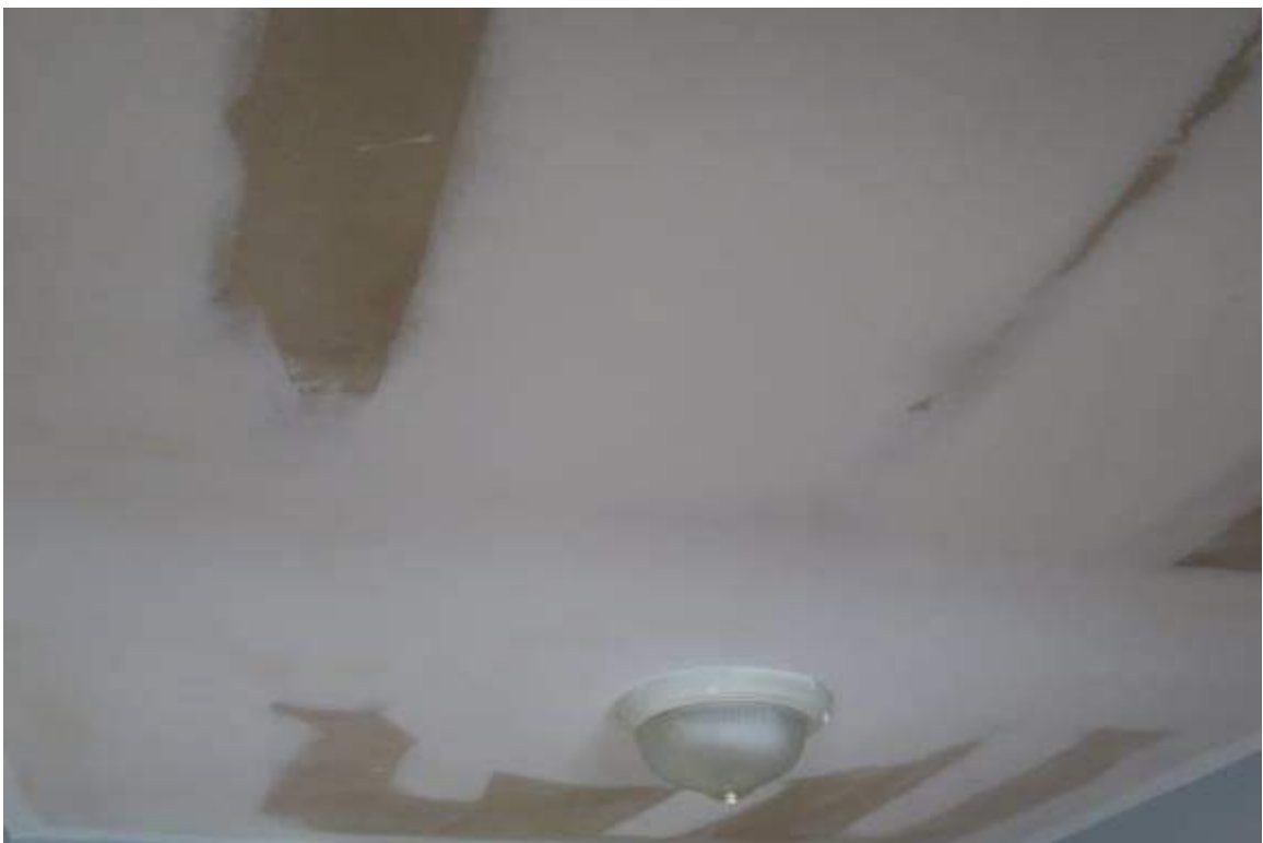
In-Process Ceiling Repair
