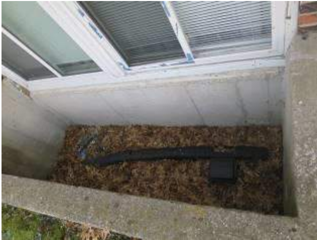
Unguarded Pit & Poor Drainage – 2644
