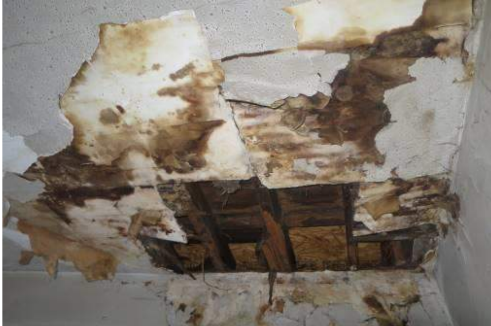
Ceiling Damage & Water Infiltration – 2651 Victor Street
