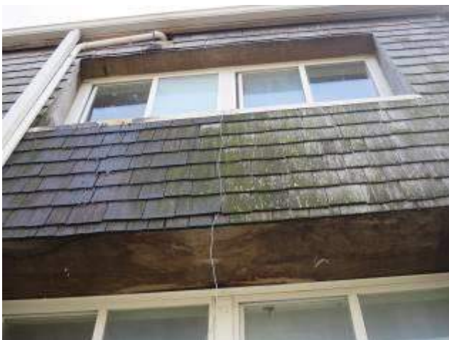
Unightly &amp; Unsafe Wiring – 2644
