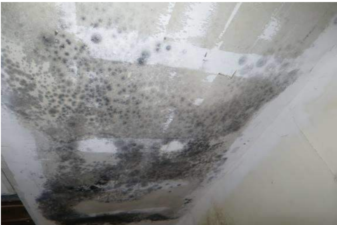
Extensive Mold Due To Water Infiltration – 2644 E 29 th Street
