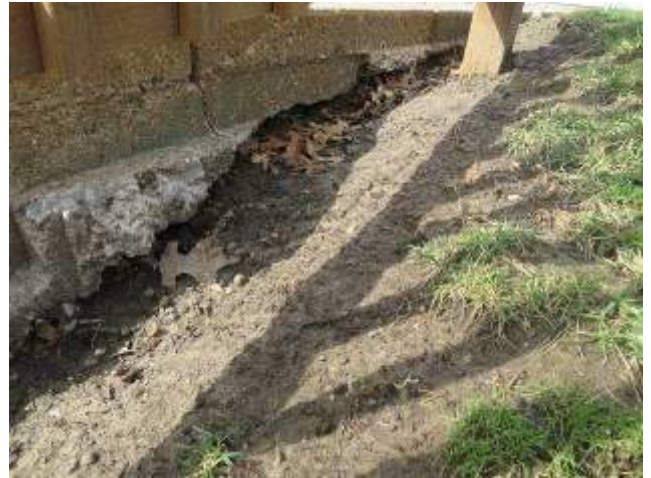
Poor Drainage &amp; Erosion – 2702
