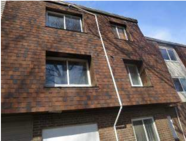
Unsightly &amp; Improper Roof Drainage – 2644
