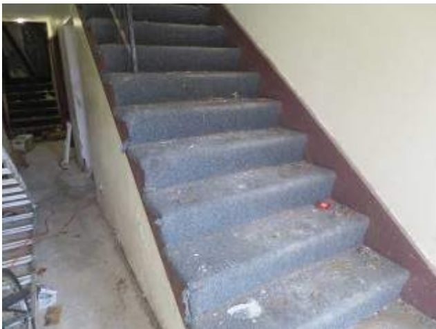
Lack Of Safety Railings On Stairway – 2644
