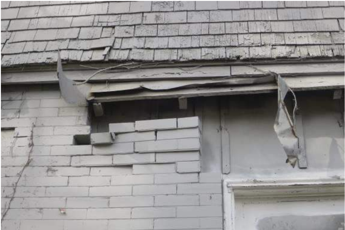
Collapsing Wall Structures – 2651 Victor Street
