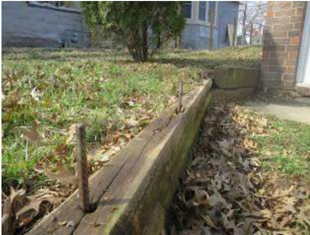
Exposed Steel Posts & Unguarded Drop Off – 2644
