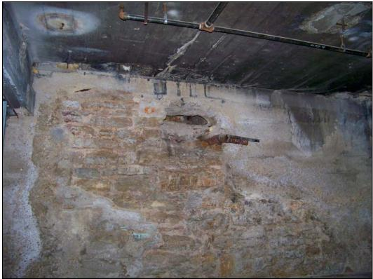
Interior – water staining, spalling of foundation wall
