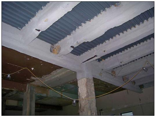
Interior – deterioration of structural beams, columns; deterioration/damage of interior finishes
