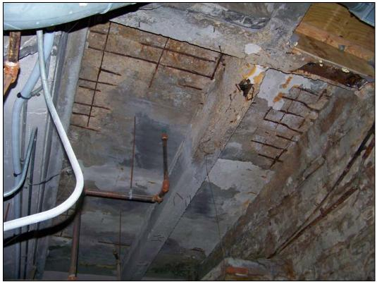
Interior – spalled concrete, exposed steel reinforcement on bottom side of elevated sidewalk over vault
