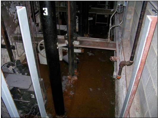
Interior – standing water at bottom of elevator shaft
