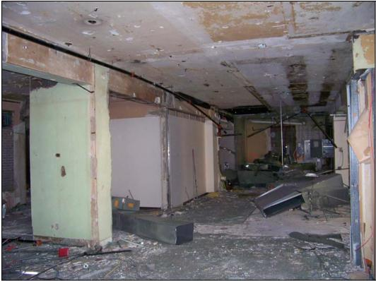
Interior – debris; disconnected HVAC, plumbing systems; lack of operable life safety systems
