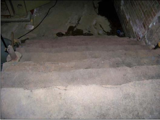
Interior – deteriorated steps with no handrail in lower level; standing water
