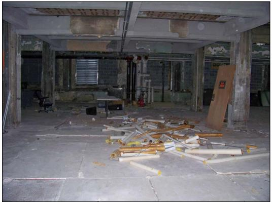
Interior - deterioration of finishes; uneven floor; debris; lack of fire suppression
