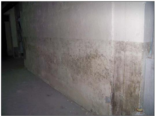
Interior – water line of flooding in lower level; water and mold damage
