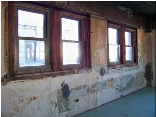
Interior – improper sealing of windows; lack/failure of finishes
