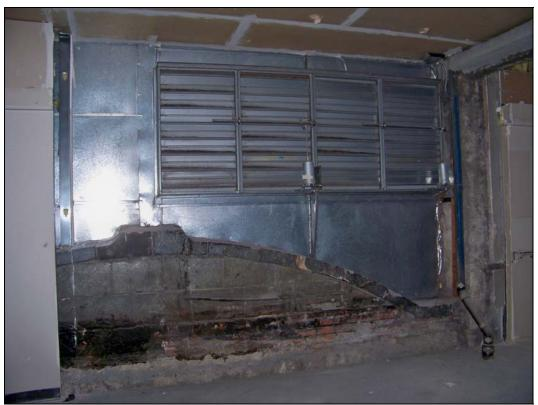
Interior – covering of gap in exterior masonry wall with sheet metal
