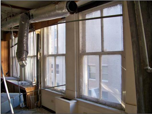
Interior – deteriorated glazing of original steel framed windows; broken glass panes
