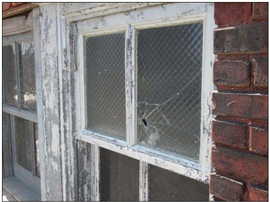
West façade – broken window panes; failure of finishes
