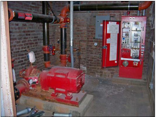
Interior – nonfunctioning fire pump, corroded
