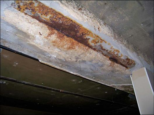
Interior – delamination of structural beam, corrosion of structural steel
