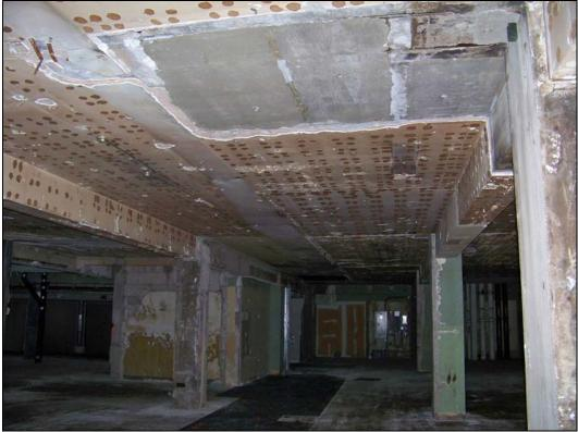
Interior – deterioration/damage of interior finishes, flooring, columns; building systems nonexistent
