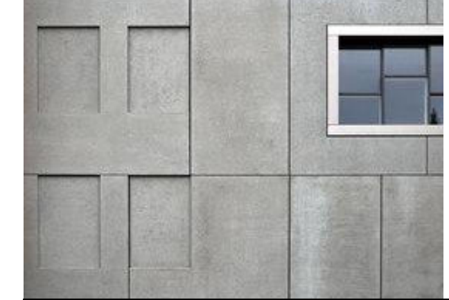
CAST-IN-PLACE CONCRETE
