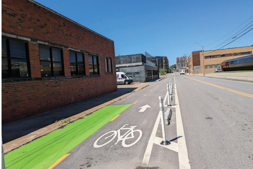
Figure 3 – Two-way cycle track using quick-build materials
