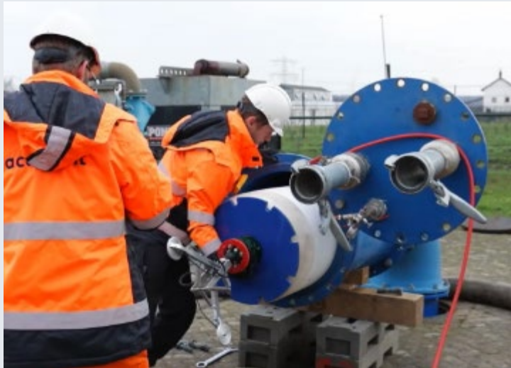
Insertion of Assessment Device into a Forcemain
