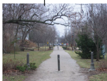
Existing Trolley Track Trail
