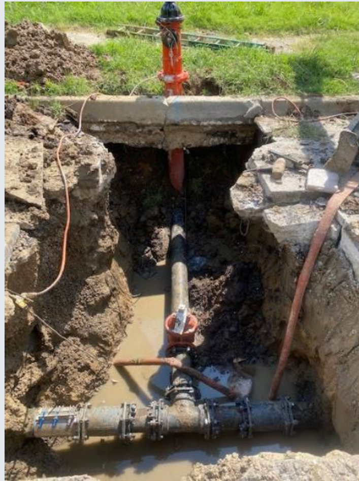
Examples of Fire Hydrant Repair Work
