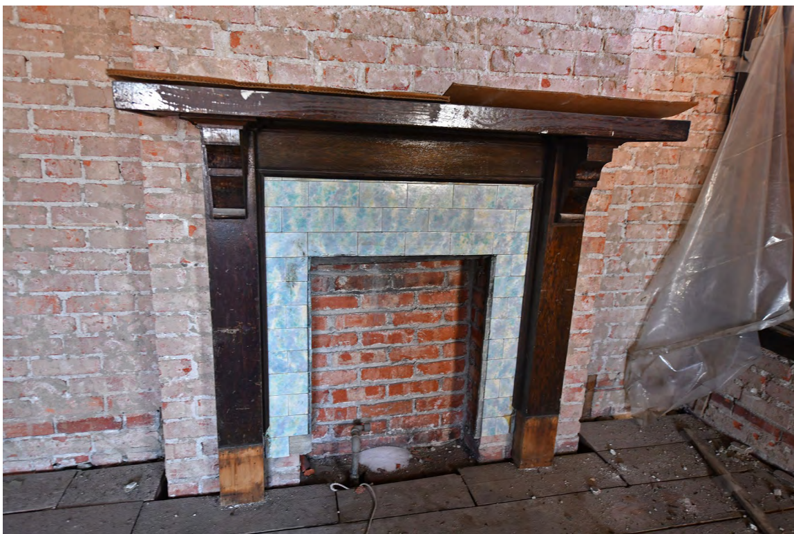
21: Interior, 3rd floor, fireplace detail, view S.
