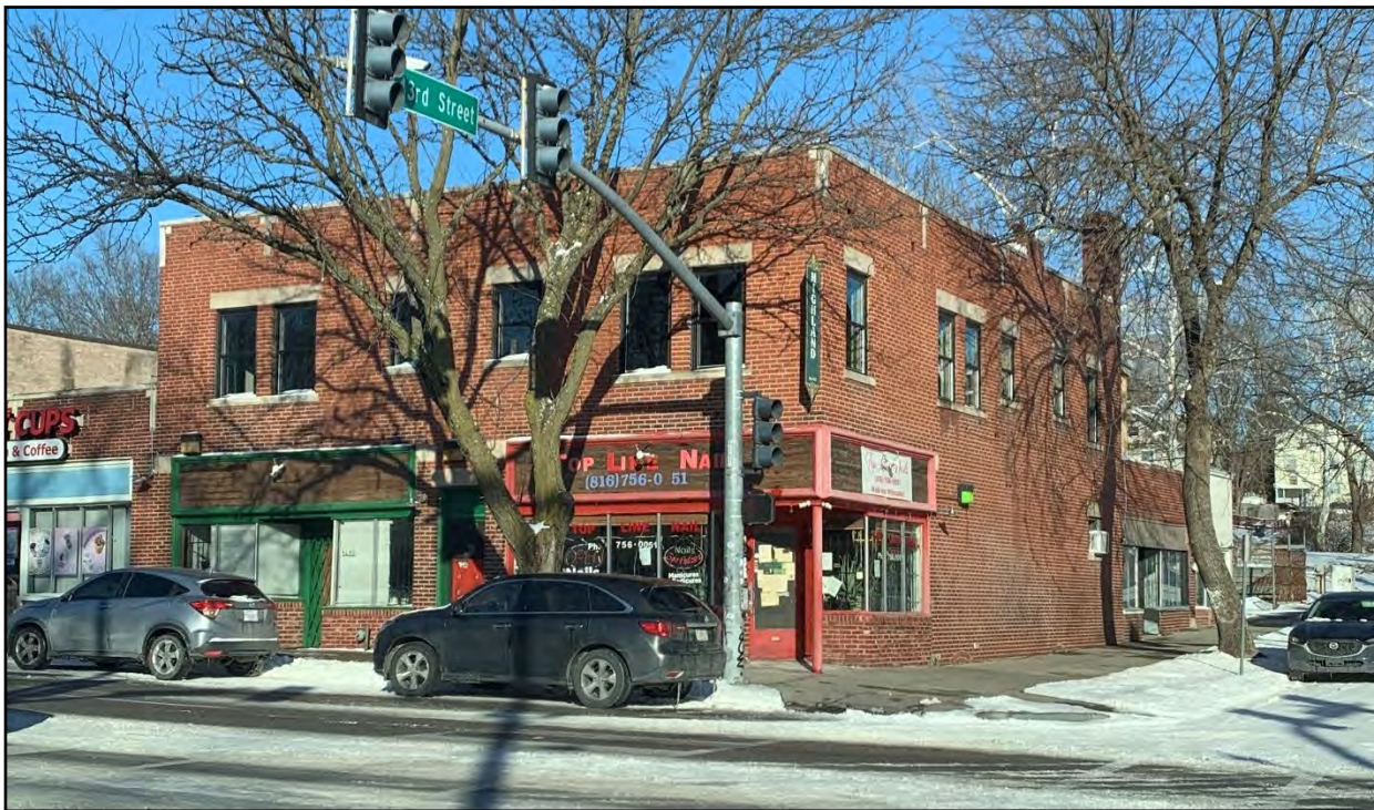
Figure 9: Building at 4245-4247 Troost Avenue (Mason Martel, 2025).
