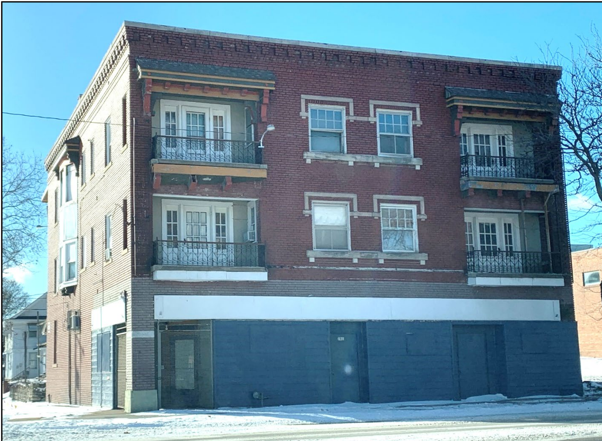
Figure 8: Building at 3942-3944 Troost Avenue (Mason Martel, 2025).
