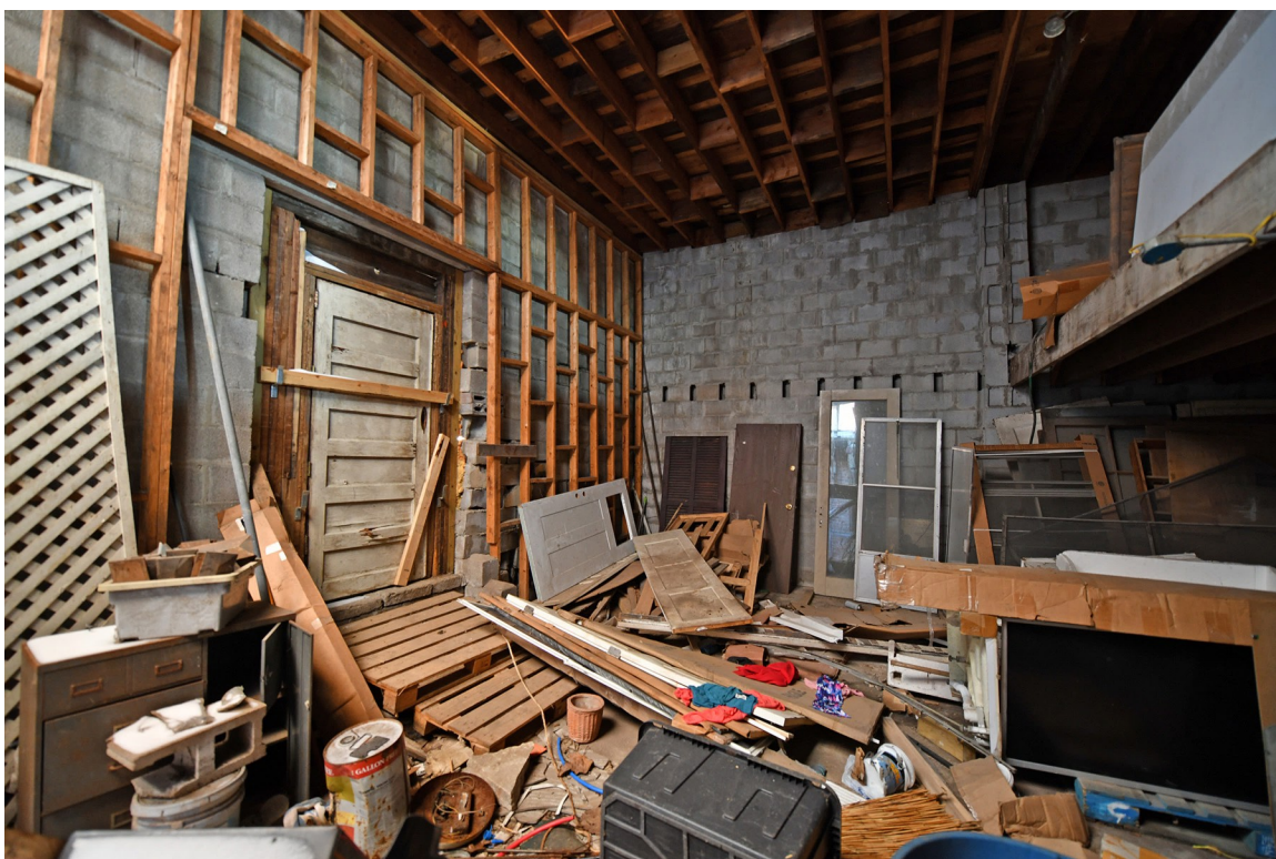
12: Interior, non-historic addition, view NE.
