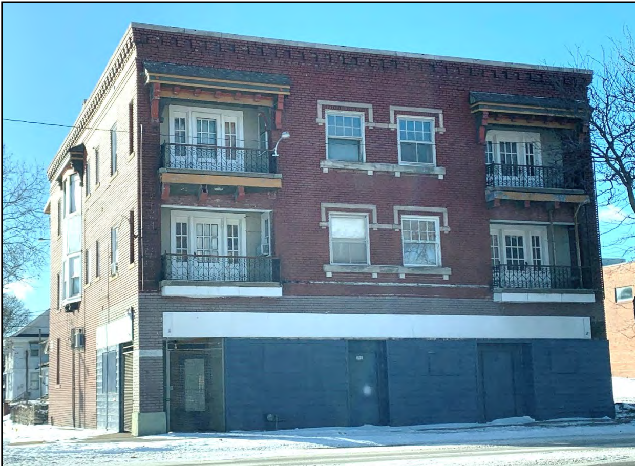
Figure 8: Building at 3942-3944 Troost Avenue (Mason Martel, 2025).
