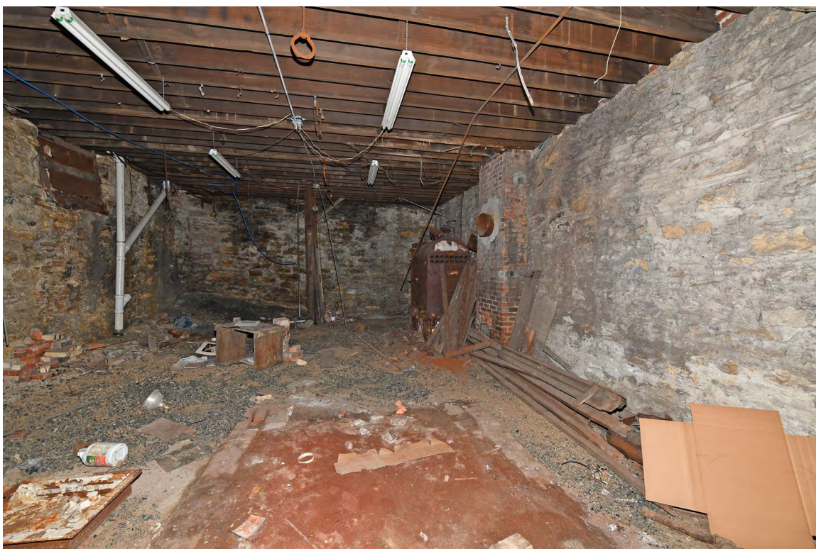
22: Interior, basement, north half, view E.
