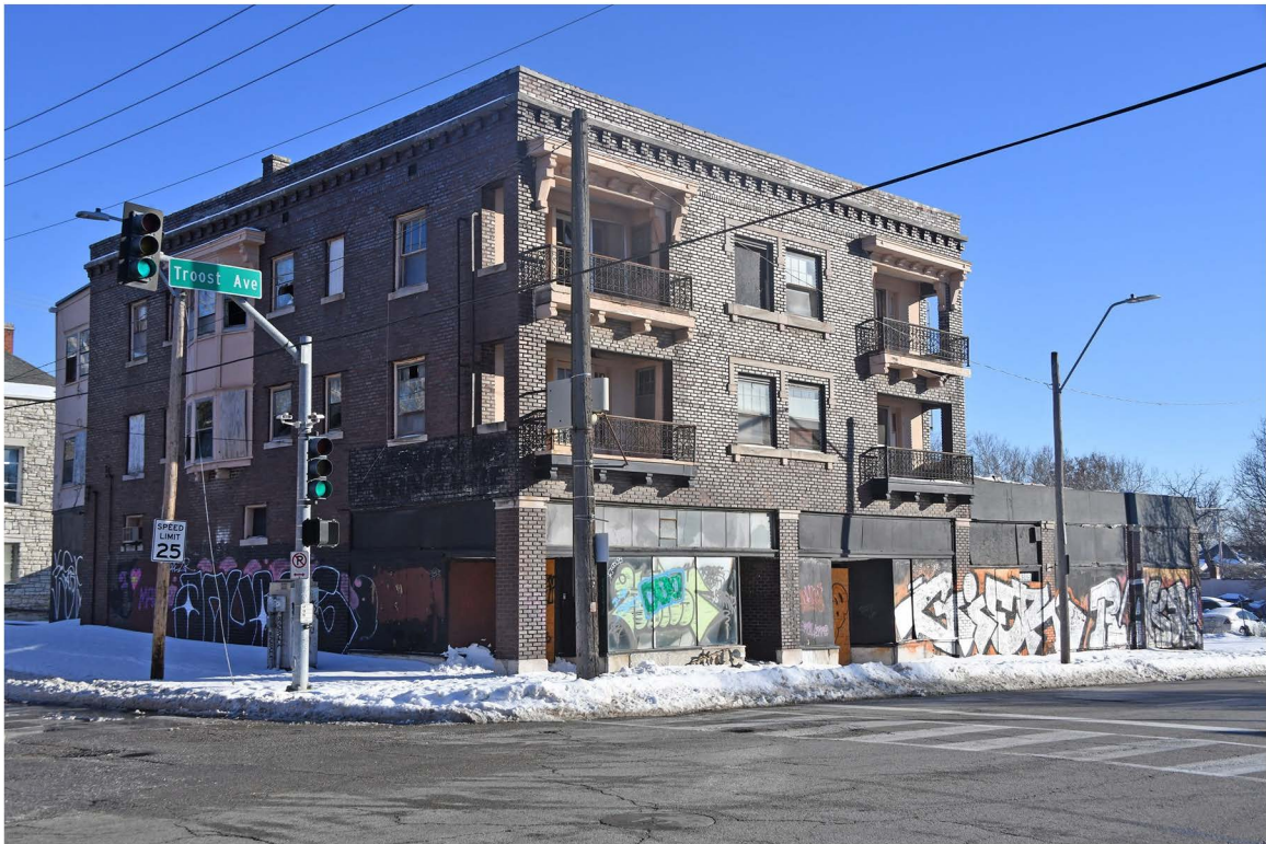
01: Exterior, northwest corner, view SE.
