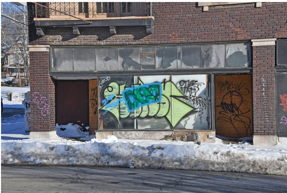
03: Exterior, west elevation, north storefront, view E.
