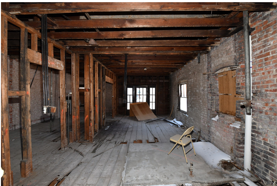
20: Interior, 3rd floor, apartment, view W.
