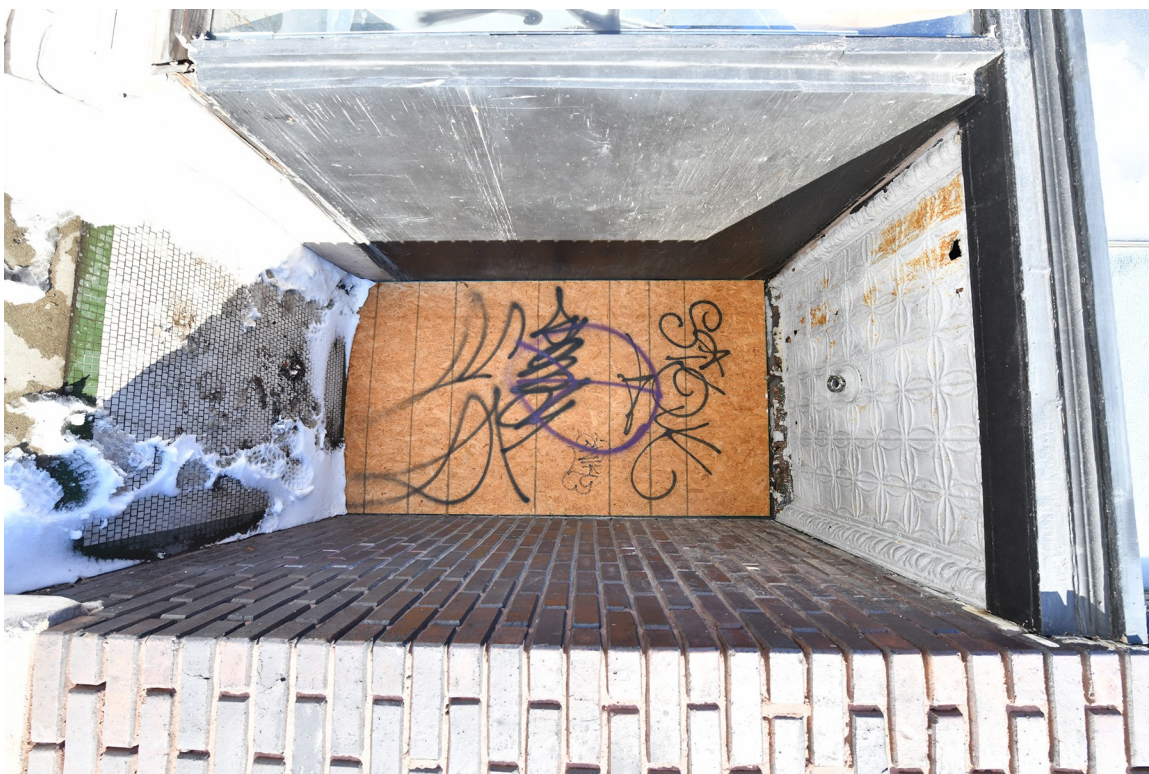
04: Exterior, west elevation, apartment entrance, view E.
