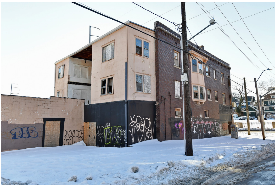
05: Exterior, northeast corner, view SW.
