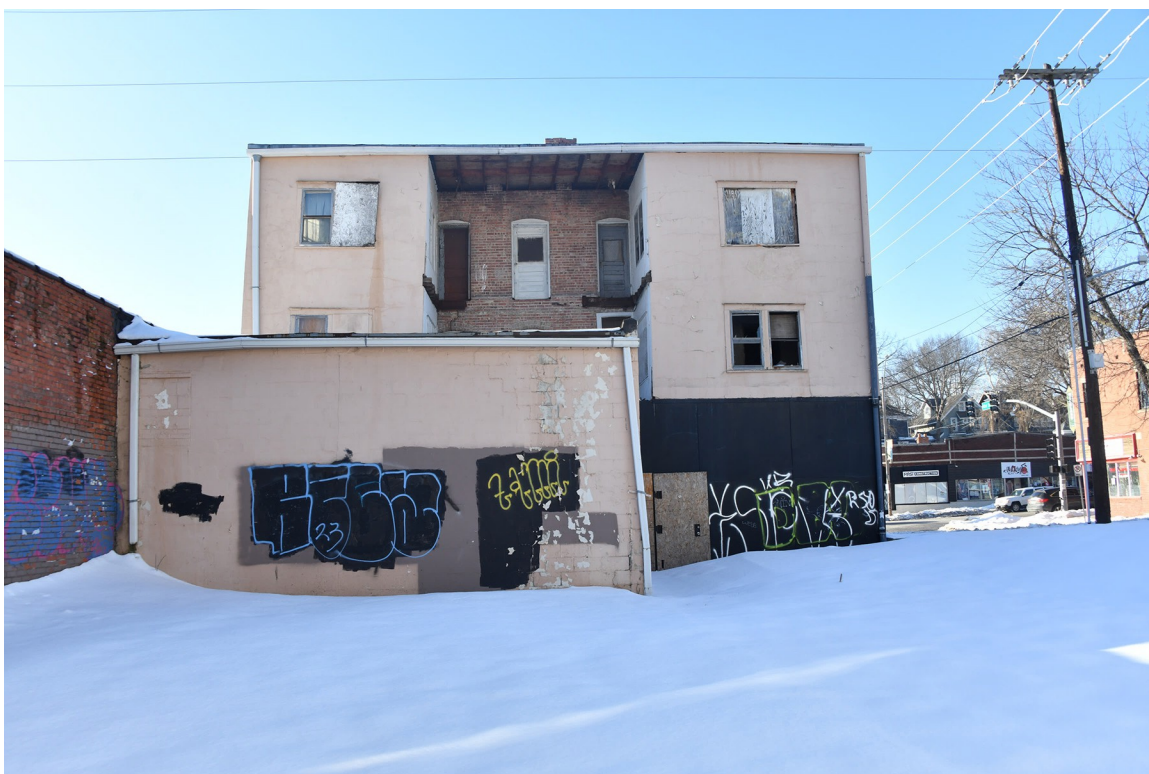
06: Exterior, east elevation, view W.
