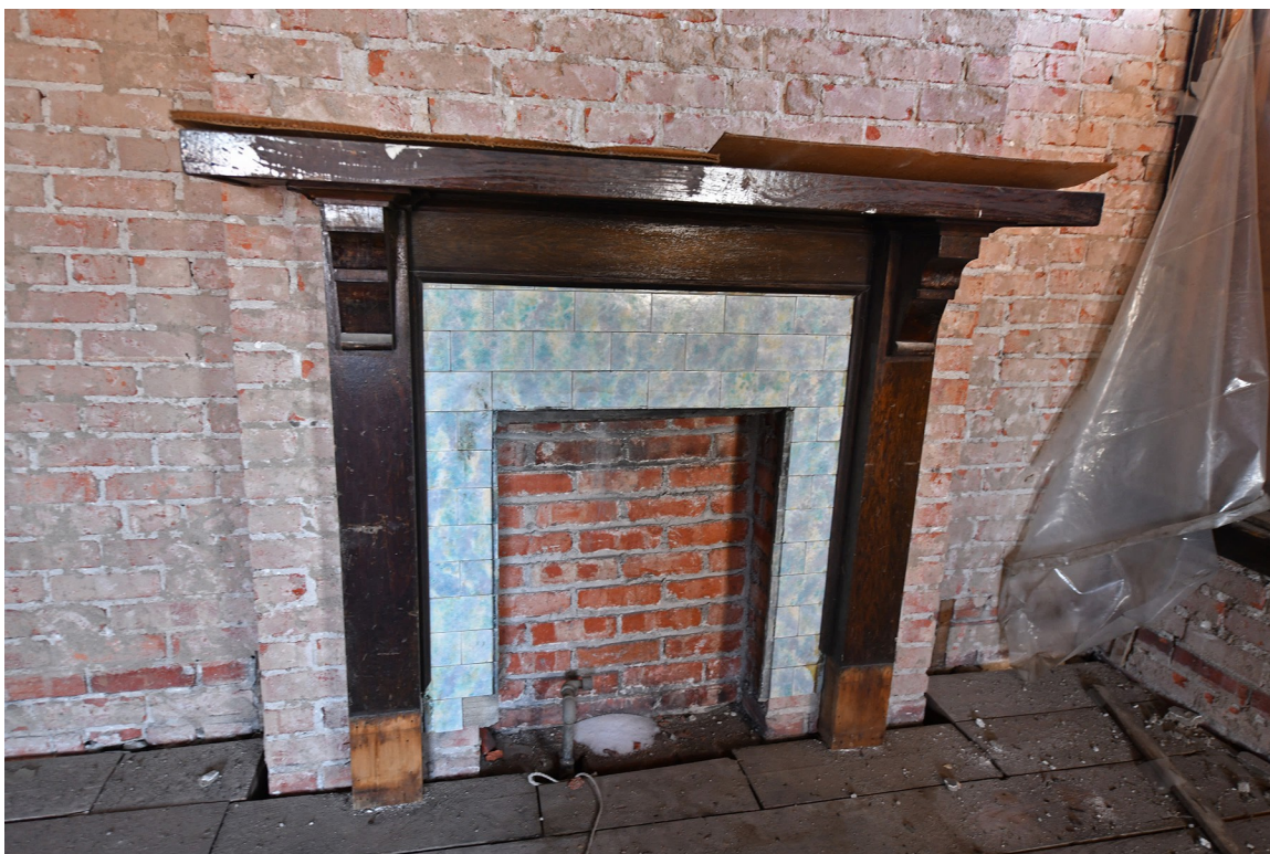
21: Interior, 3rd floor, fireplace detail, view S.
