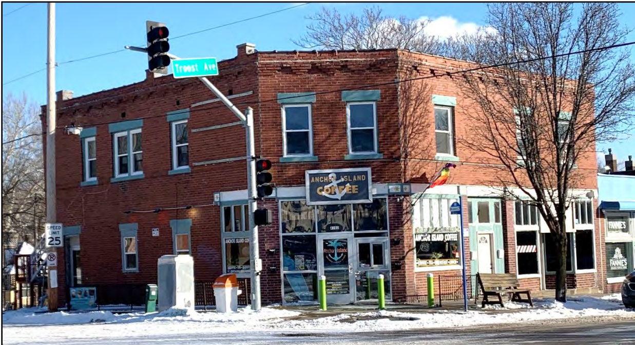
Figure 10: Building at 4101-4103 Troost Avenue (Mason Martel, 2025).
