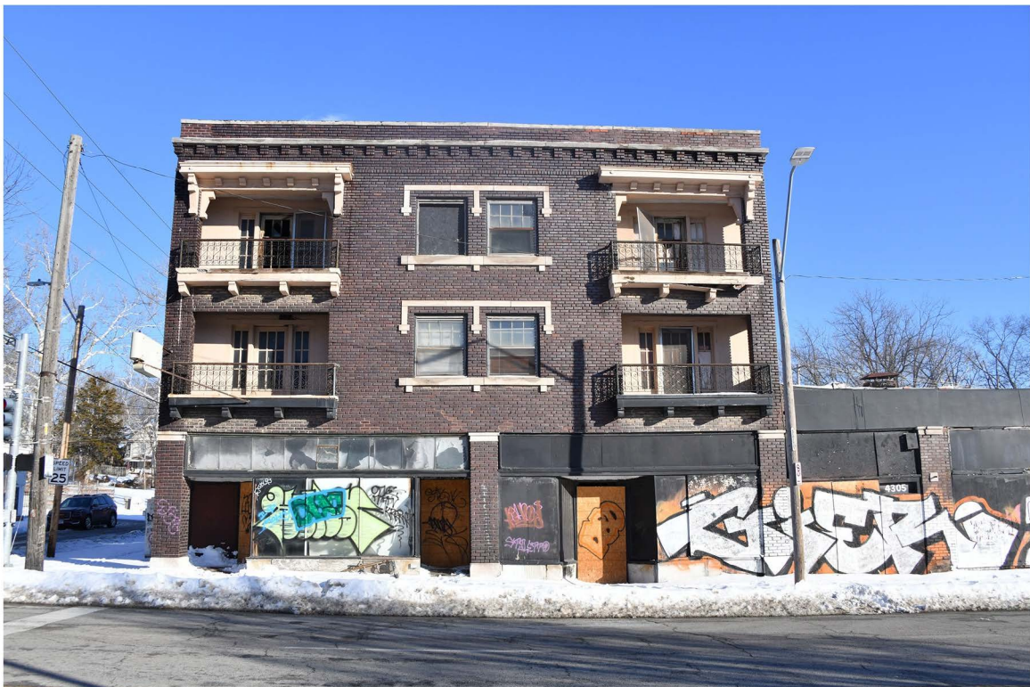
02: Exterior, west (primary) elevation, view E.
