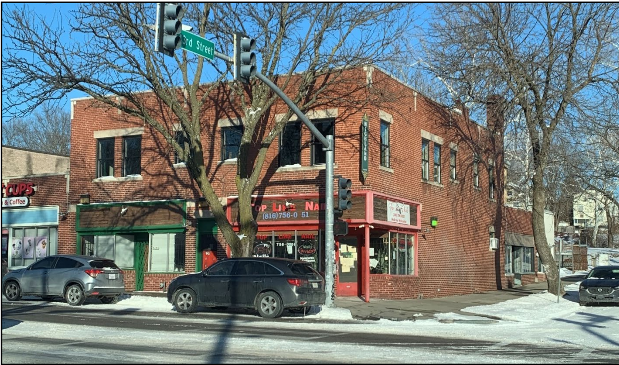
Figure 9: Building at 4245-4247 Troost Avenue (Mason Martel, 2025).
