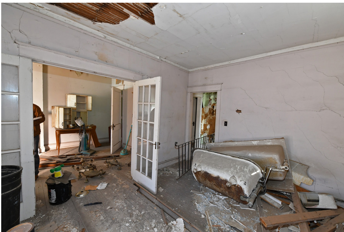
16: Interior, 2nd floor, apartment bedroom, view NE.
