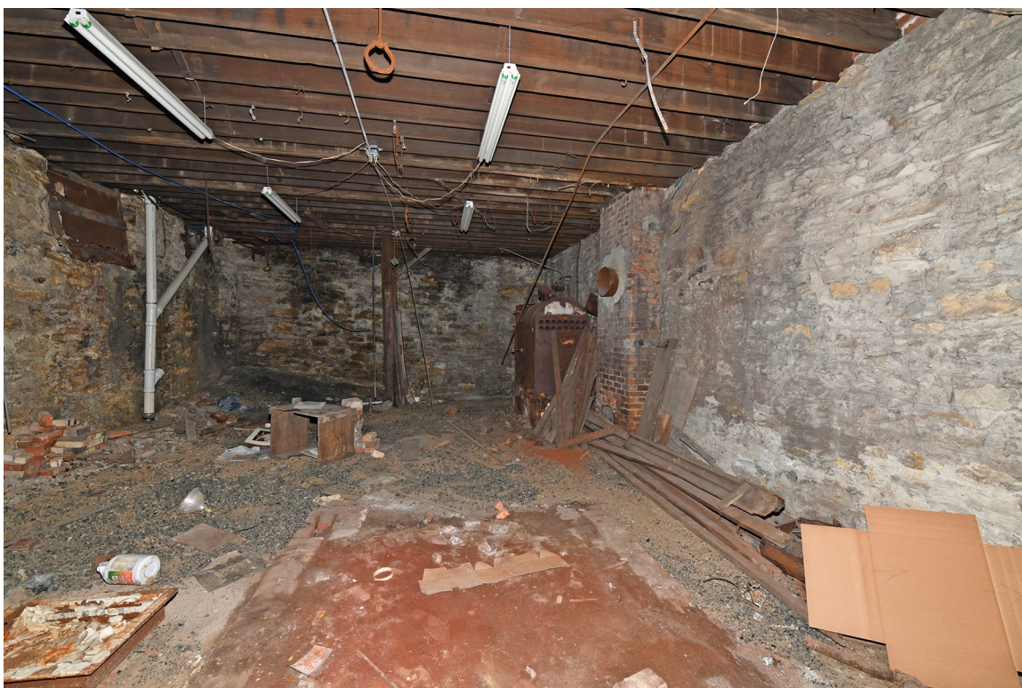
22: Interior, basement, north half, view E.
