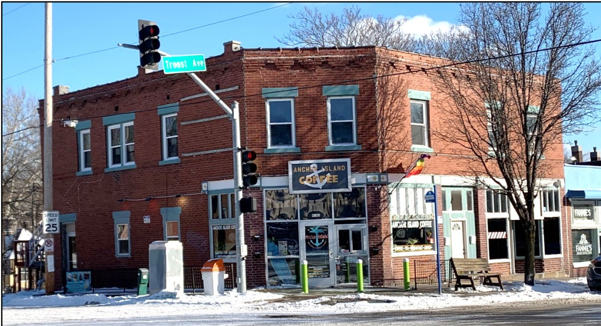
Figure 10: Building at 4101-4103 Troost Avenue (Mason Martel, 2025).
