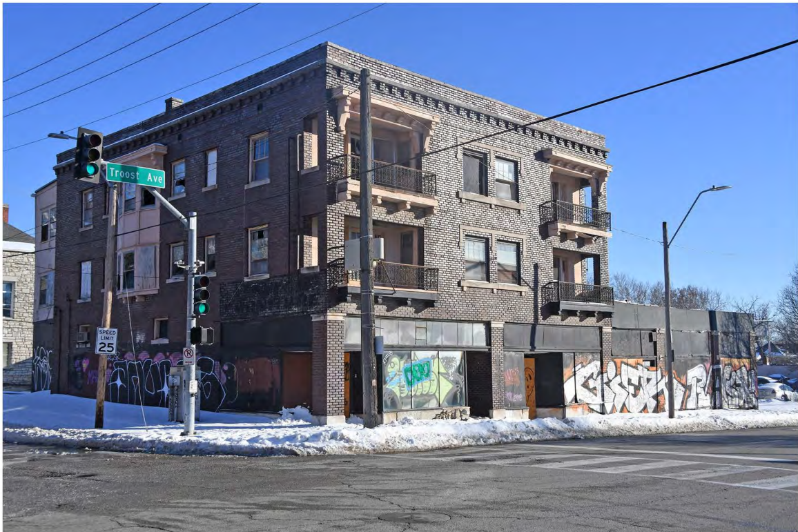
01: Exterior, northwest corner, view SE.
