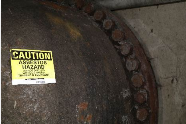
Deteriorated Twin 60-Inch Force Main Pipes
