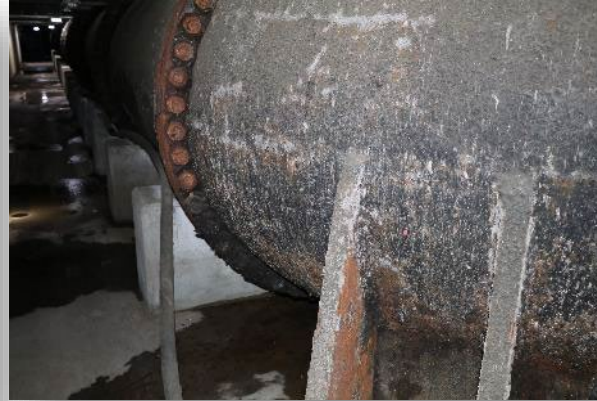
Deteriorated Twin 60-Inch Force Main Pipes
