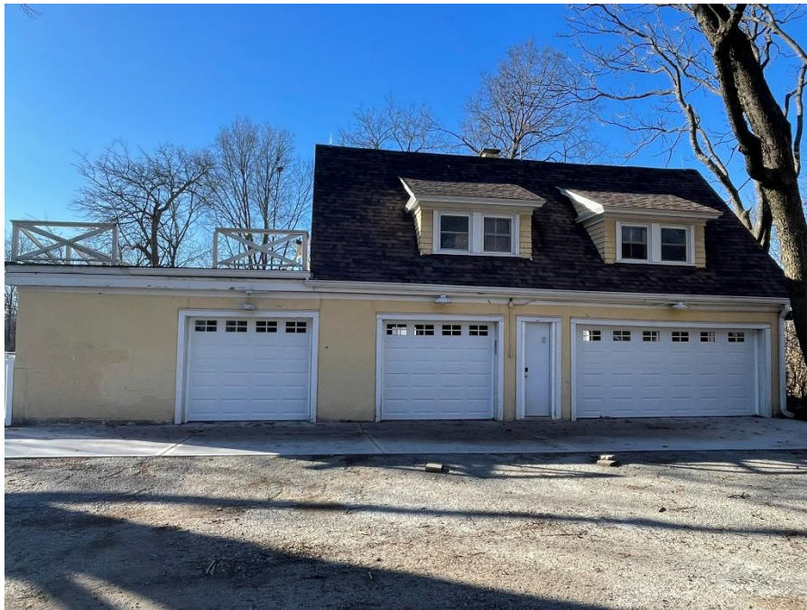
Resource No. 2 Carriage House (East Façade)
