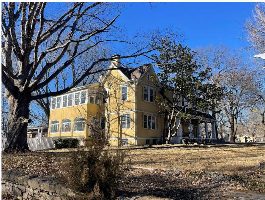
Resource No. 1: Main House (South Façade)
