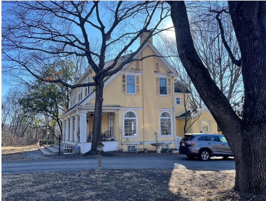
Resource No. 1: Main House (North Façade)
