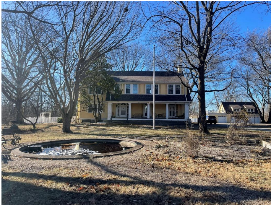
Resource No. 1: Main House (East Façade)
