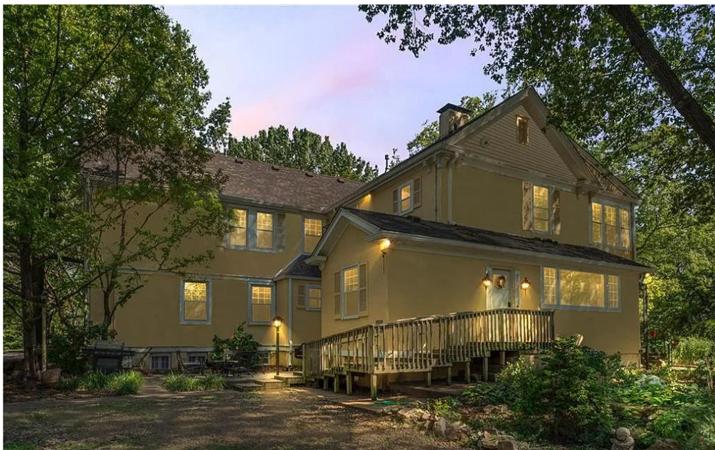
Resource No. 1 Main House (West Façade)
