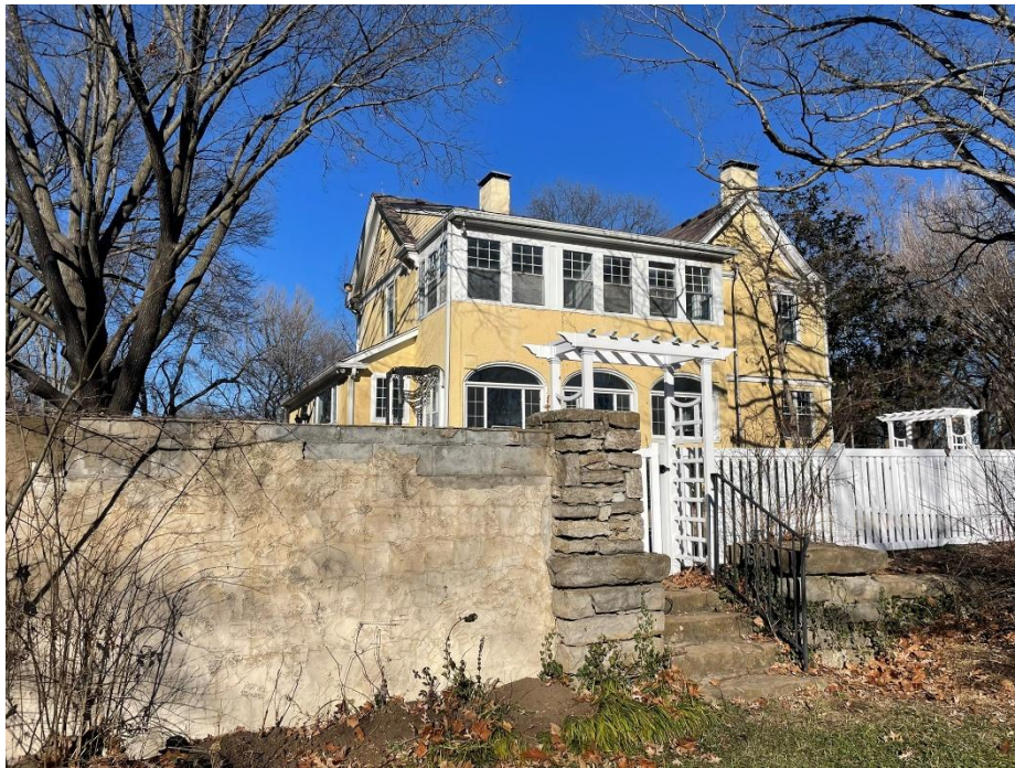
Resource No. 1: Main House (South Façade)
