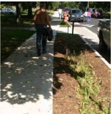
In residential areas, include vegetated swales in lieu of enclosed stormwater pipe systems along the roadways.
