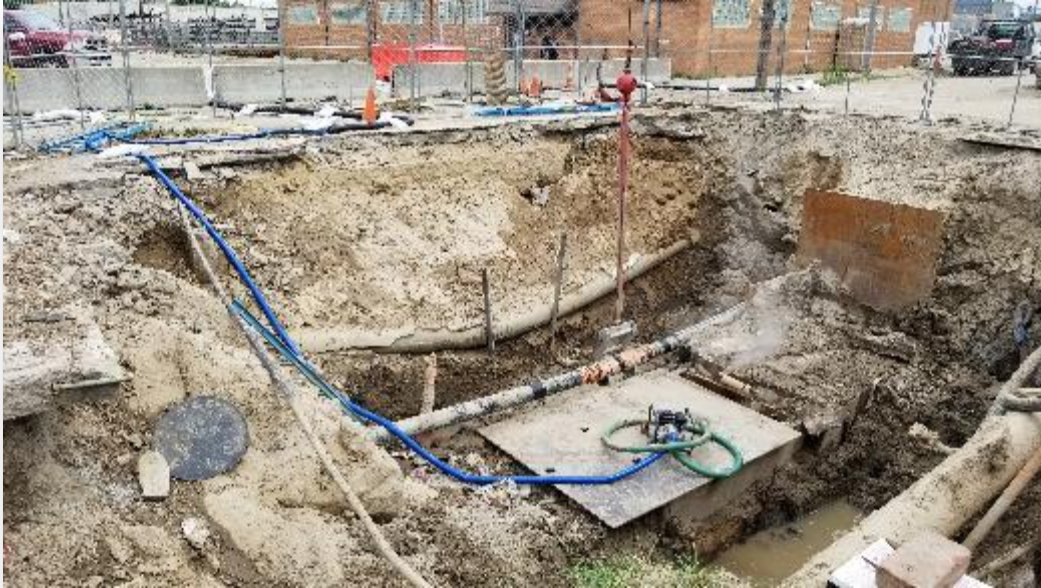
Emergency 18-inch Sewer Repair at 1700 Guinotte Avenue
