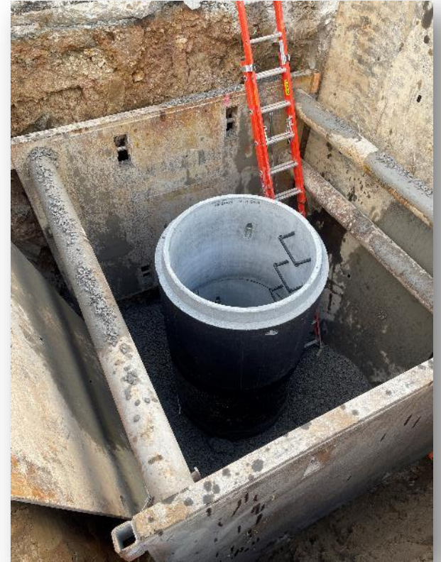
Sewer Manhole Replacement
