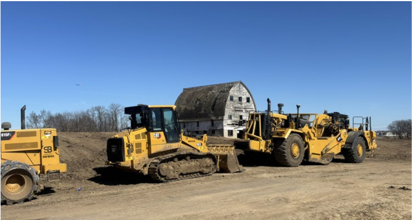
Grading land for new subdivision, January 2026.
