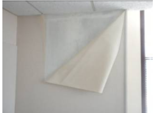
Delaminating Wallcovering
