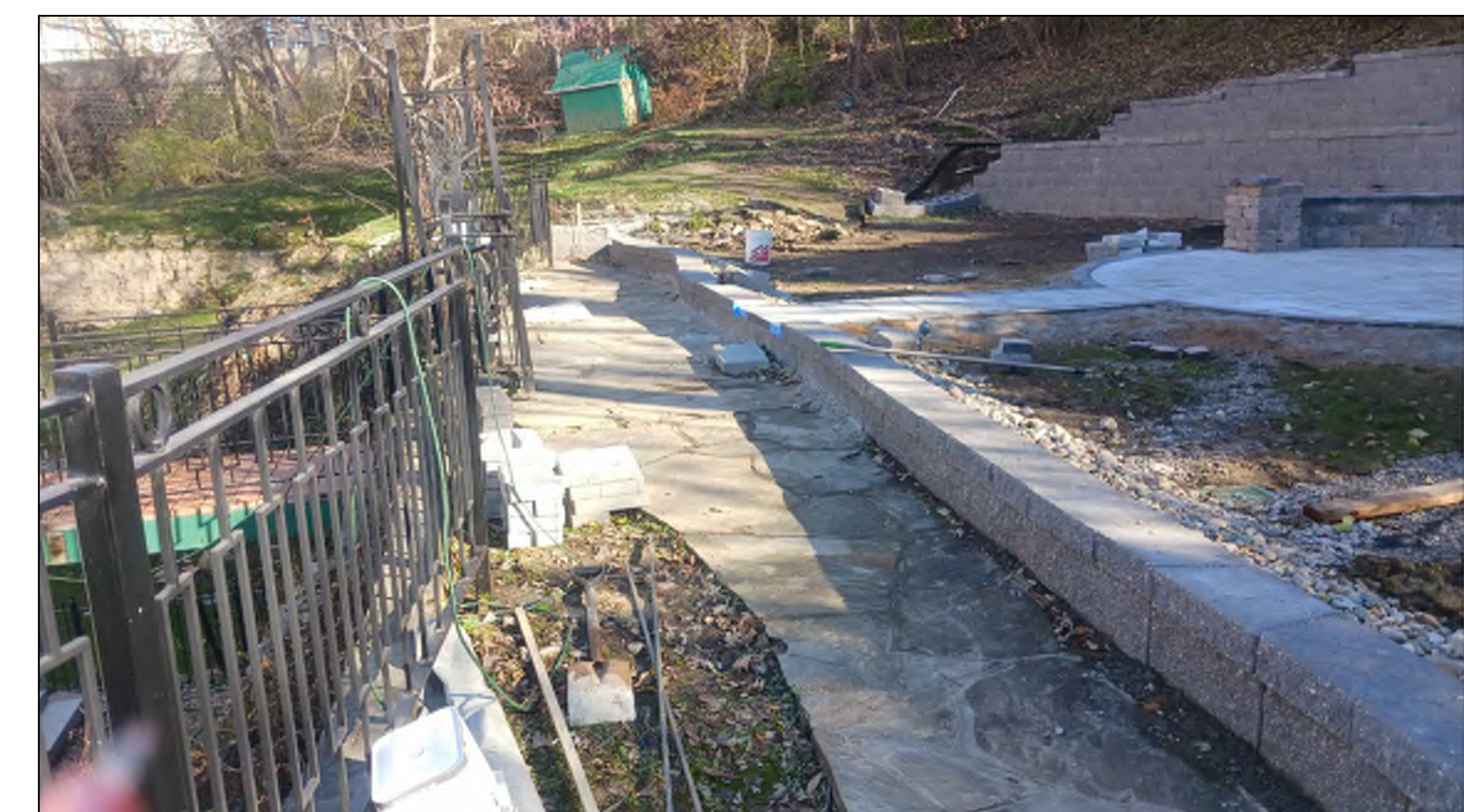
RETAINING WALL (SHORT SECTION)
