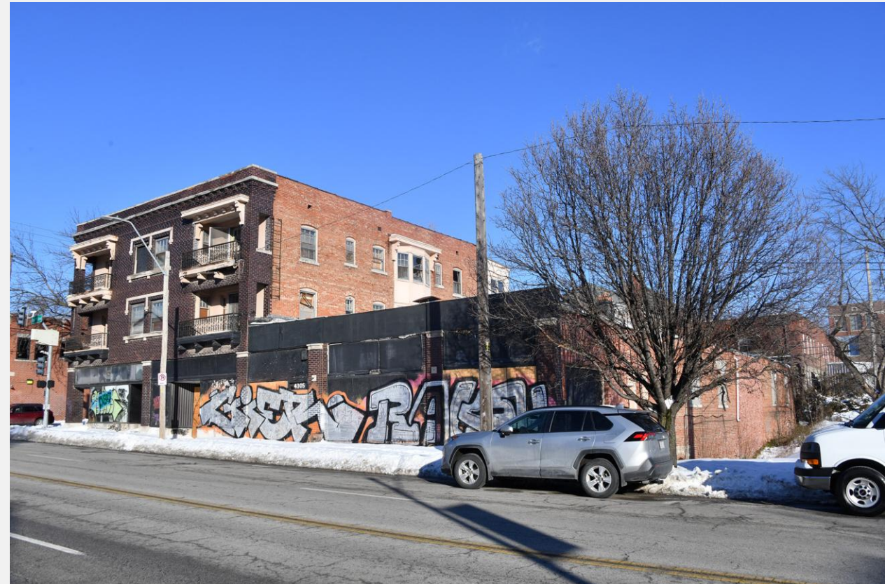
View from Troost Ave (West)
