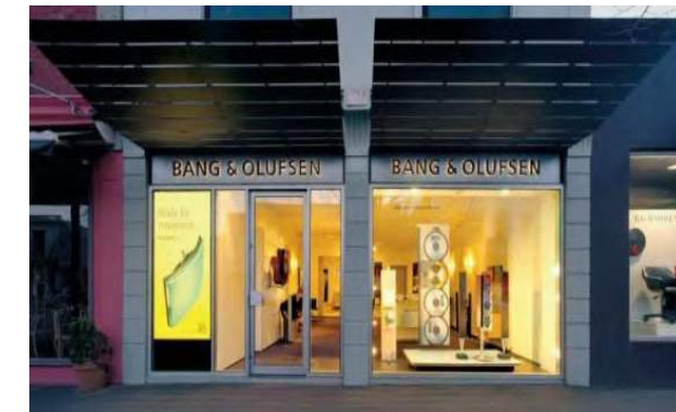
Canopy Canopy is 10'-0" or higher above walkway Transparent Entrance Entry accent element.
