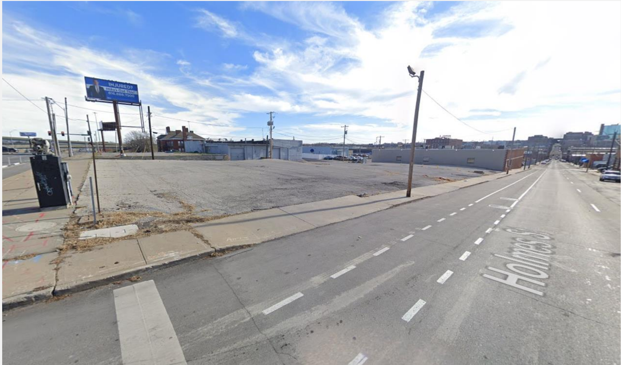
View towards site going south on Holmes St (Dec 2023)
