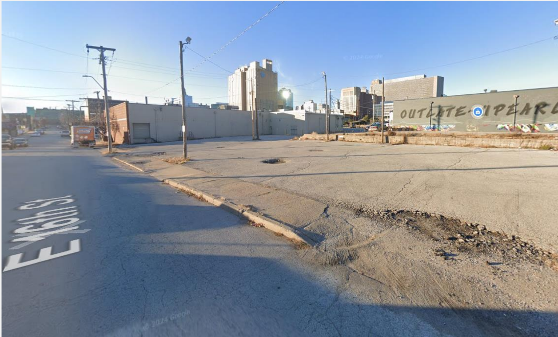
View from 16 th St & Charlotte St towards site. City-owned parking lot to be used and existing alley to access parking garage.
