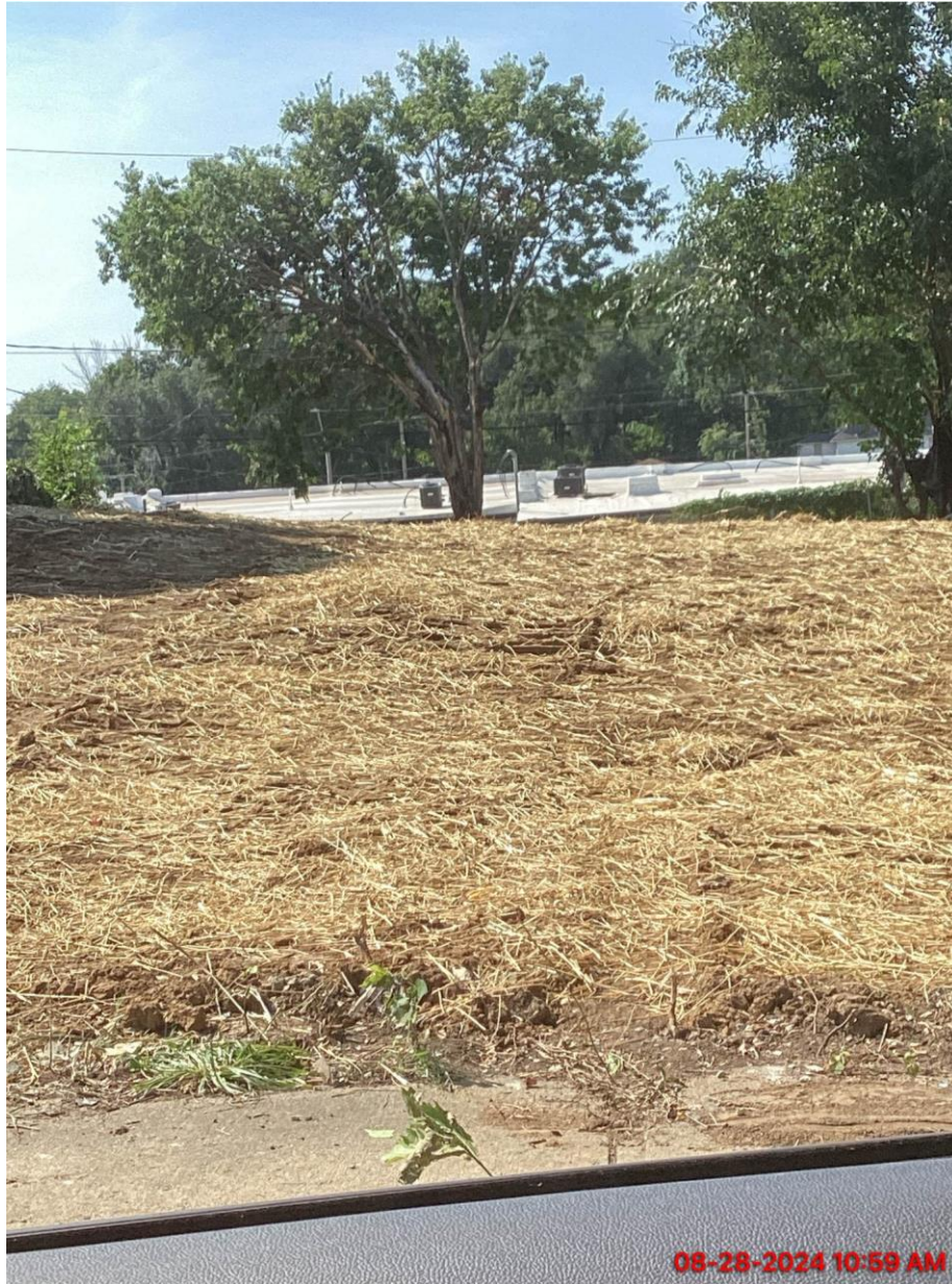
Image from Demolition Final Inspection – August 28, 2024
