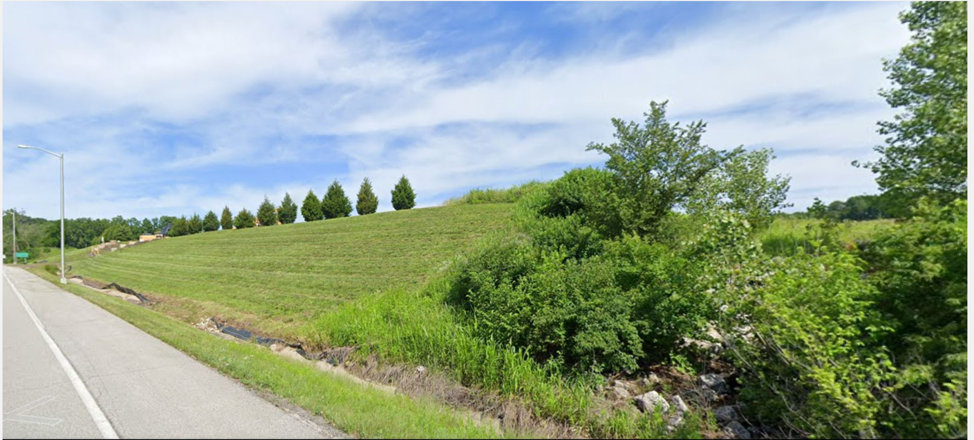
View from NE Service Road
