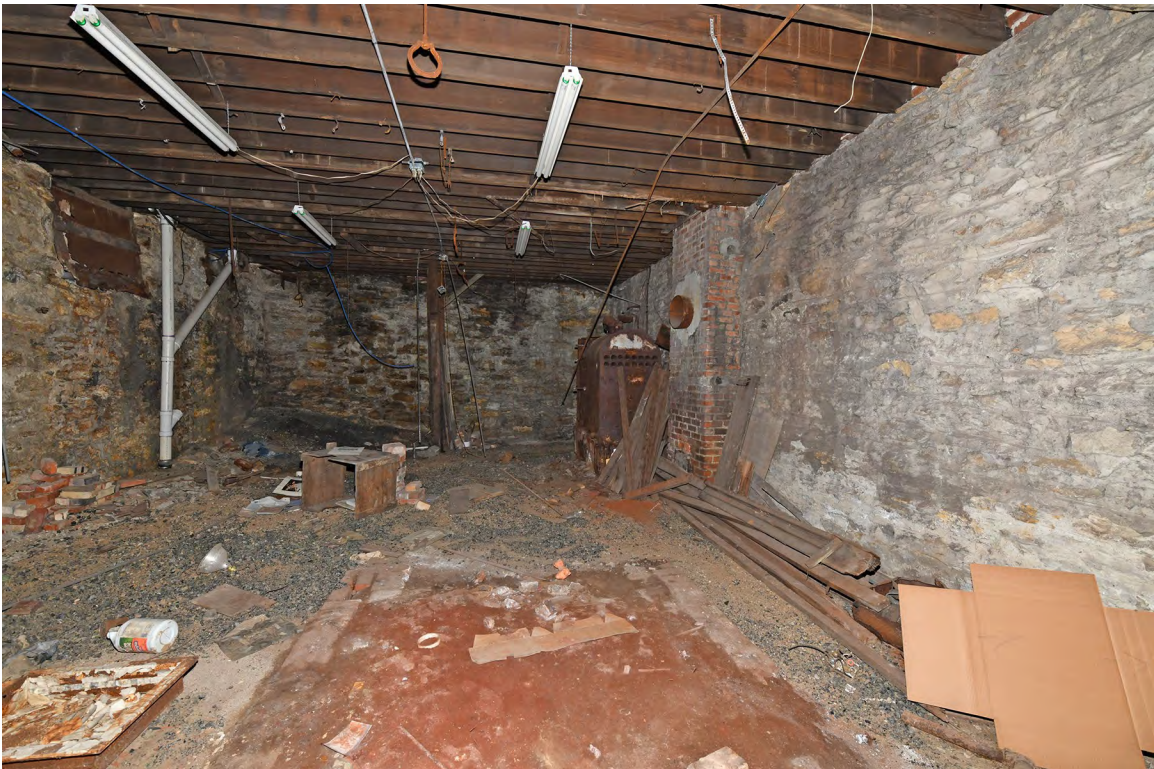
22: Interior, basement, north half, view E.
