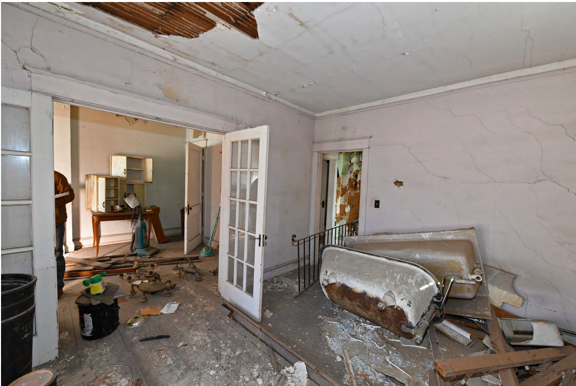
16: Interior, 2nd floor, apartment bedroom, view NE.
