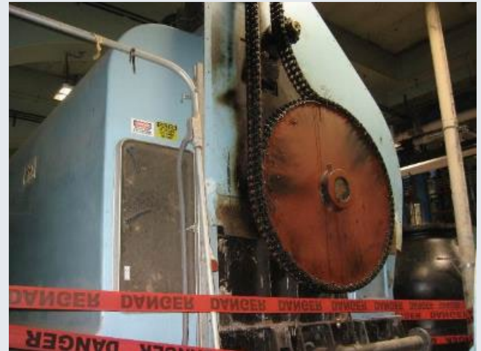
Housing for the River Intake Traveling Screens
