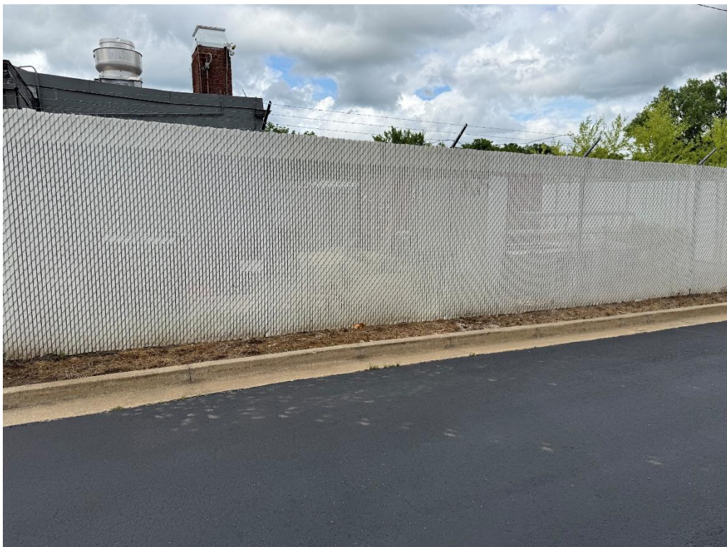
Existing screen fence viewed from adjacent property.
