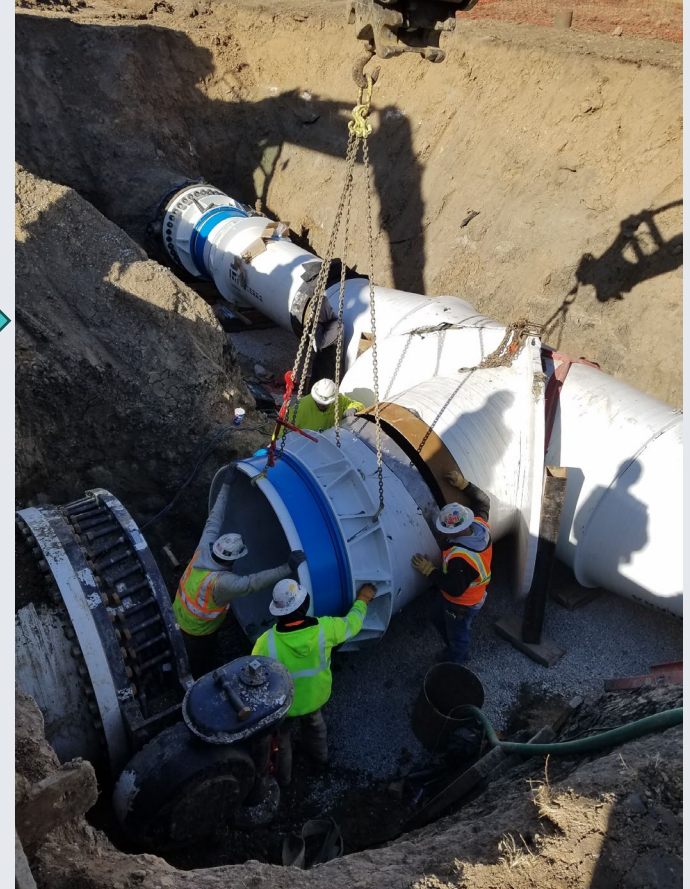
Emergency Transmission Repairs
