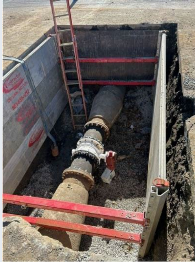
Replacement of a Ball Valve with a Butterfly Valve
