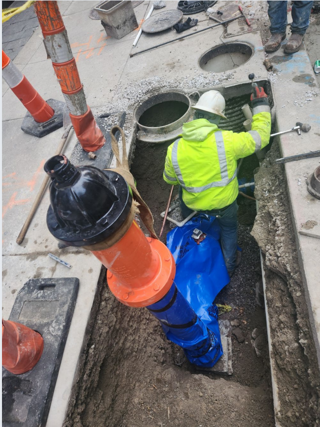
Emergency Distribution Repairs
