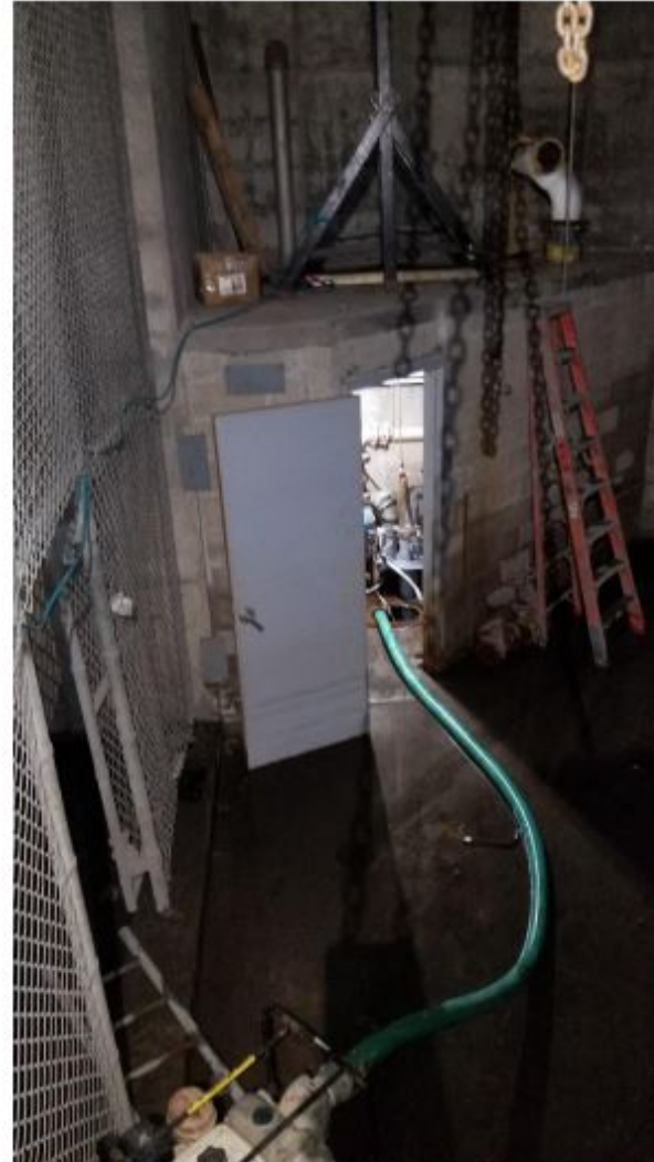
Fig. XX SE Fan room sump pump repair underway
