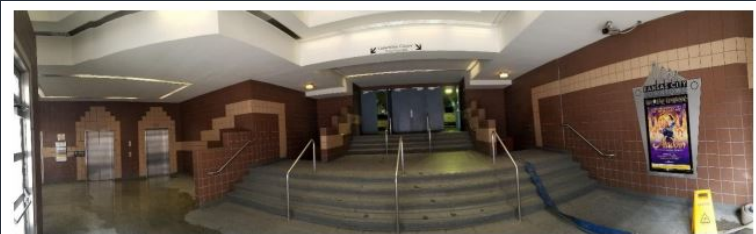
Fig. XX No discernable emergency lights at south street indoor entrance
