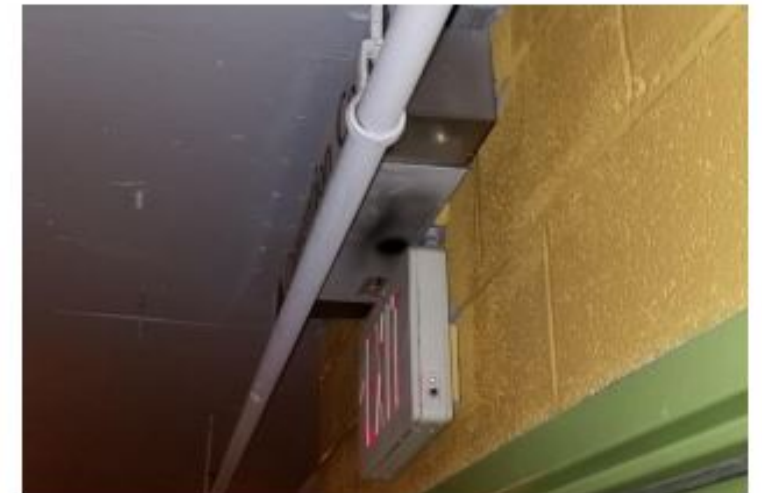
Fig. XX Non-working emergency light above exit
