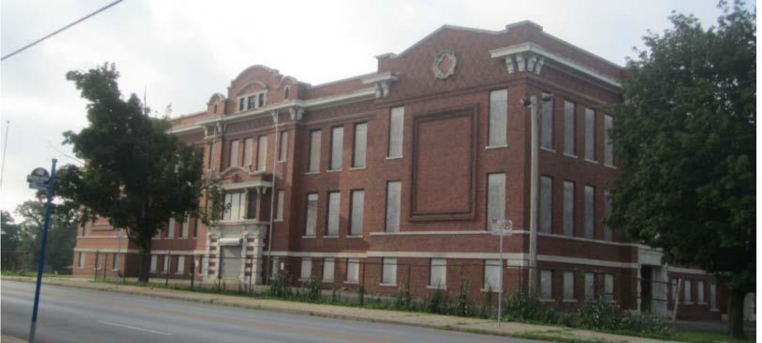
Figure 3 - Former Greenwood School.
