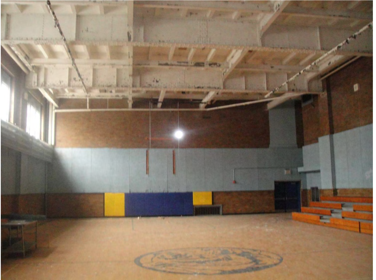
Photo 64 – Overall view of the lower gymnasium.
