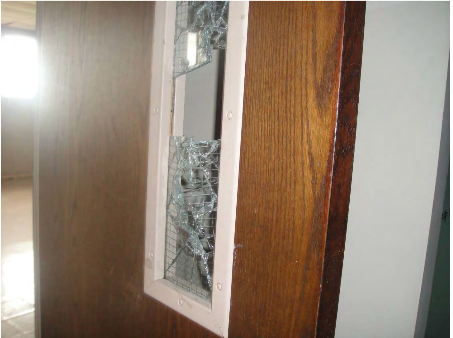
Photo 53 – Deteriorating Site Condition.
