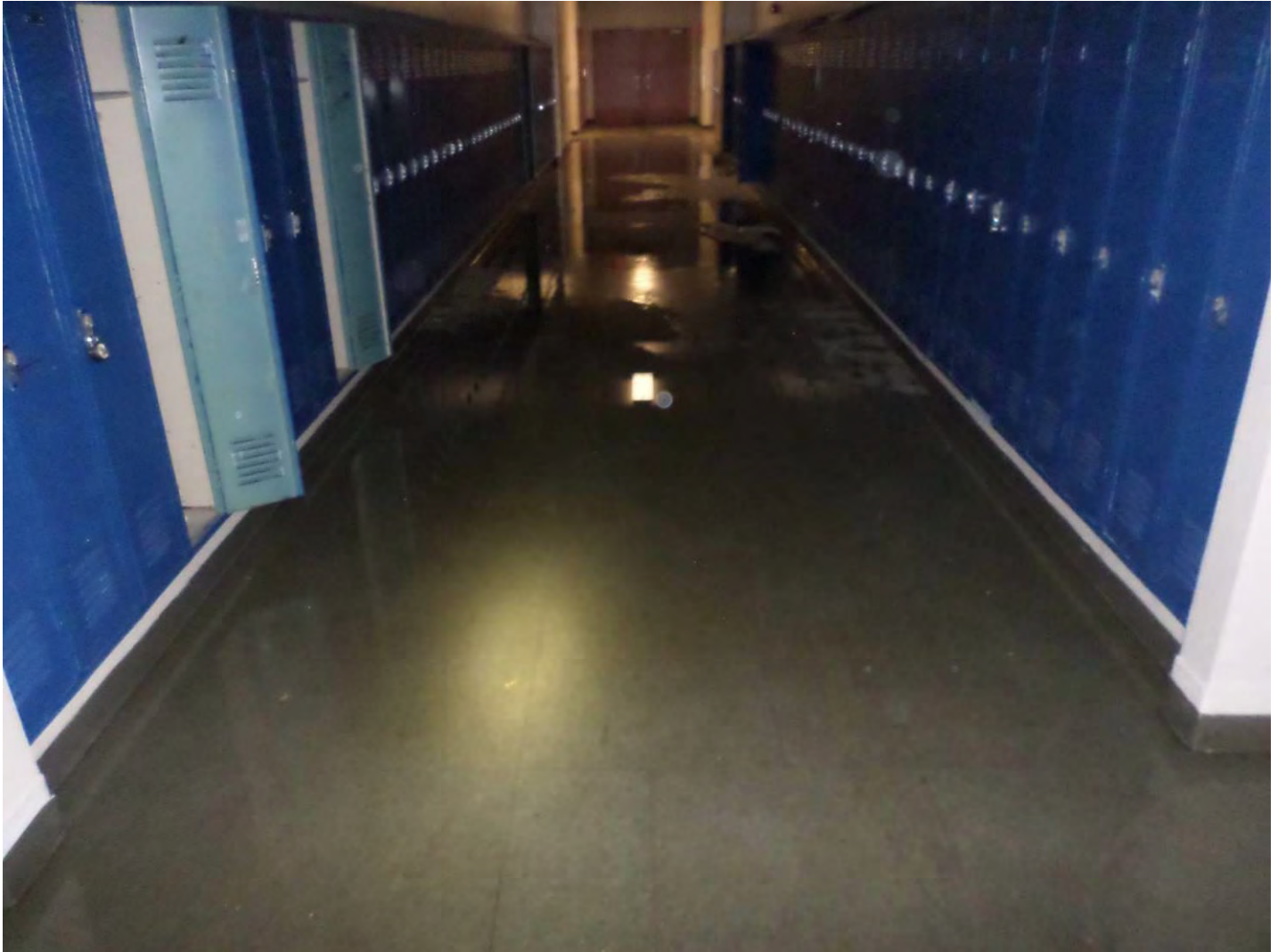
Photo 36 – Deteriorated Site Improvements. Photo courtesy property owner
