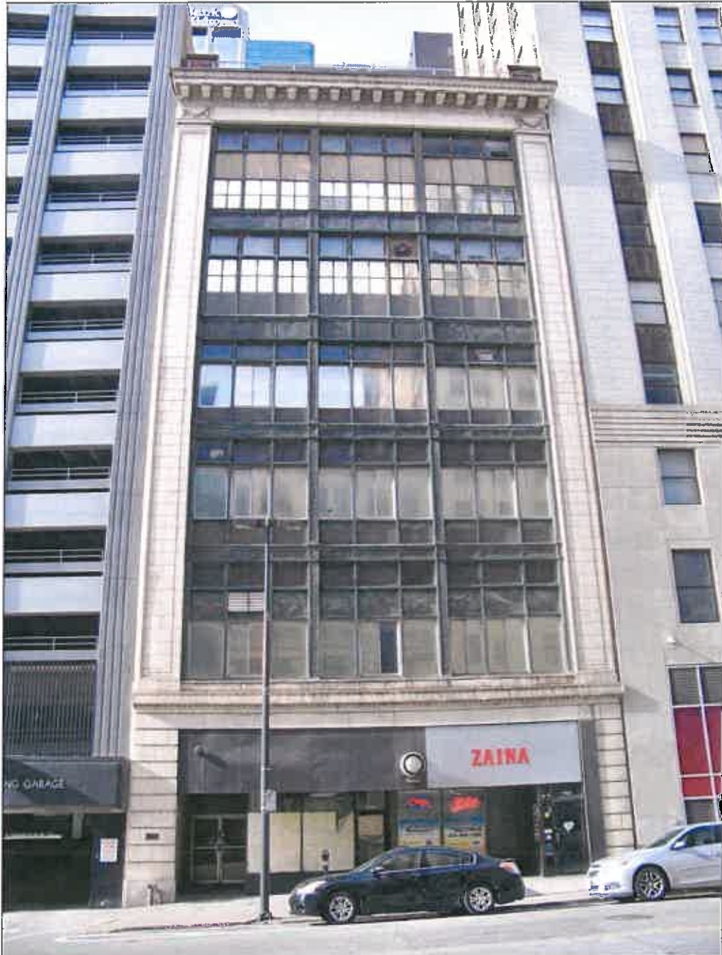
1108-1110 Grand Boulevard – East Elevation (front of building facing Grand Boulevard)
