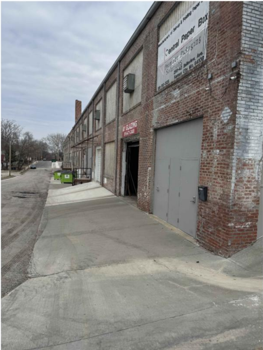
View from South looking North at building
