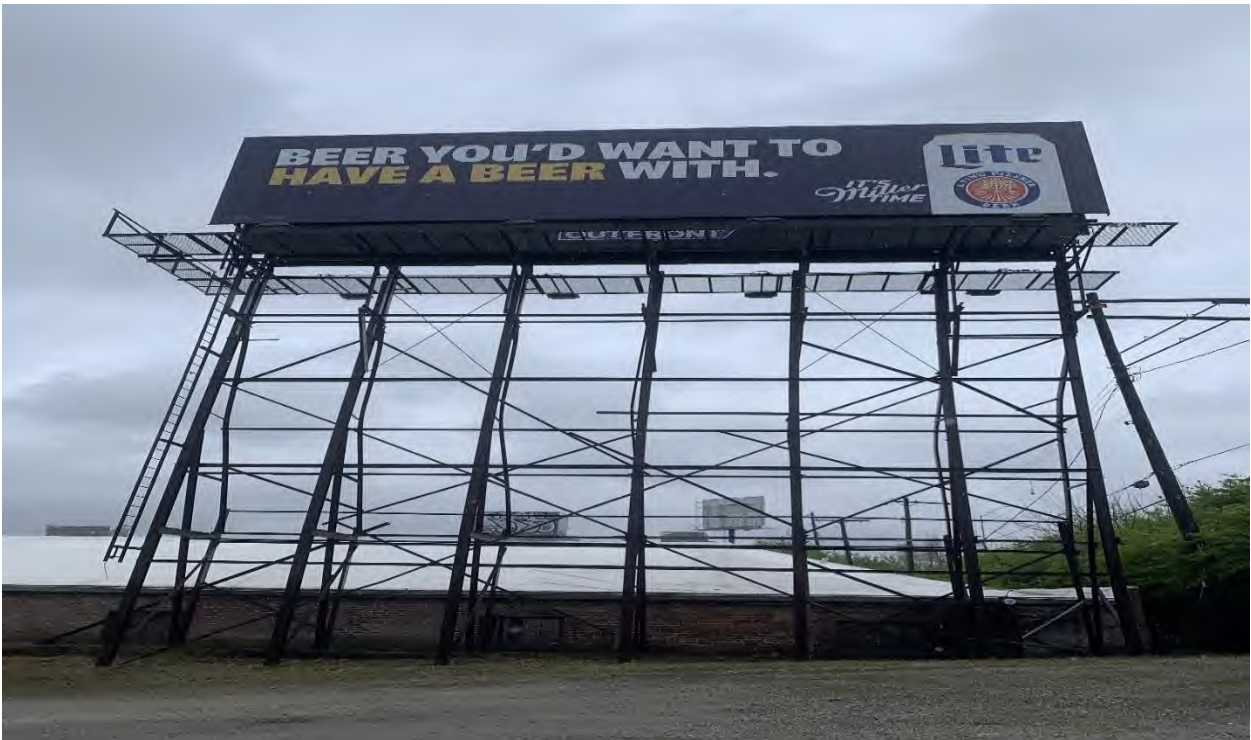
Figure 2. 17th St. and Washington. Southwest corner billboard.
