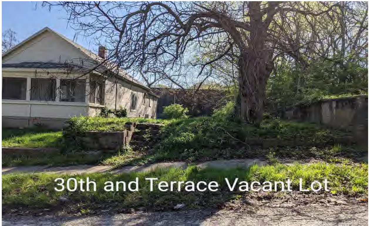
Figure 11. 3007 Terrace St. Vacant, unimproved lot.
