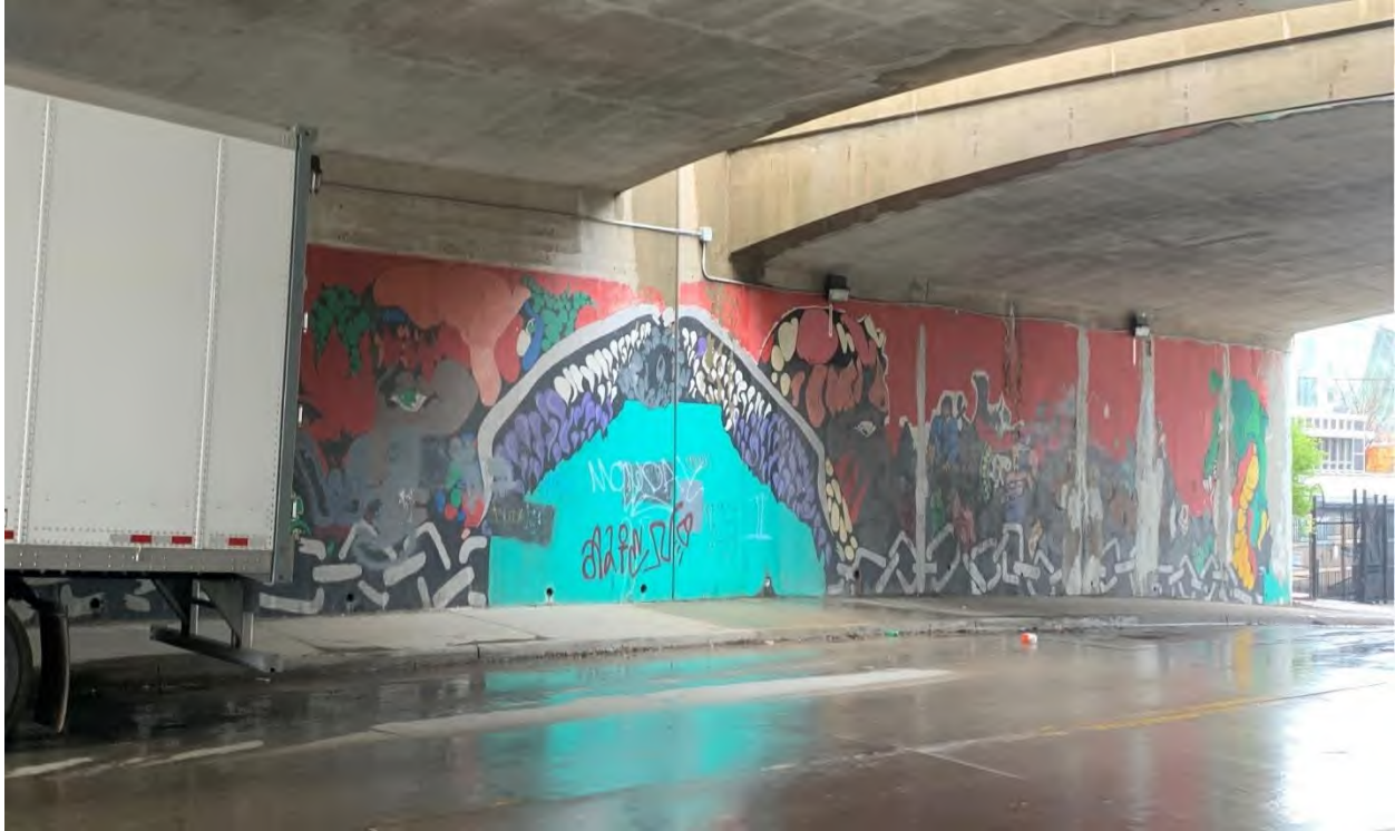
Figure 12. Underpass of 17th Street, west of Washington. Graffiti over art wall.
