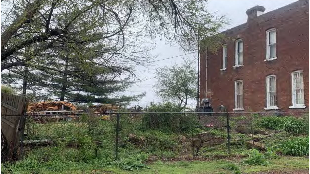
Figure 7. 802 W. 16th St. Large woodpiles in overgrown yard present a fire hazard.
