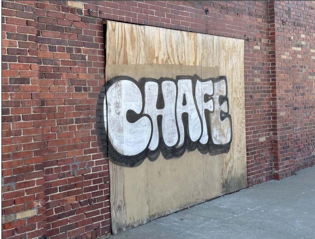
1905 Walnut Street – looking west – graffiti on east side of building
