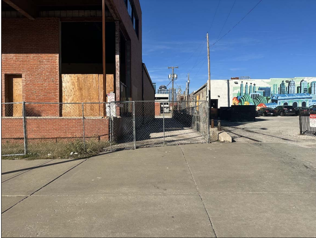
100 E. 20 th Street – looking north – narrow one-lane drive with no signage, pavement markings
