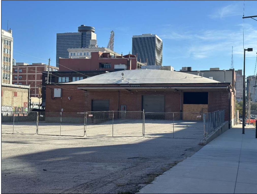
100 E. 20 th Street – looking south at north elevation
