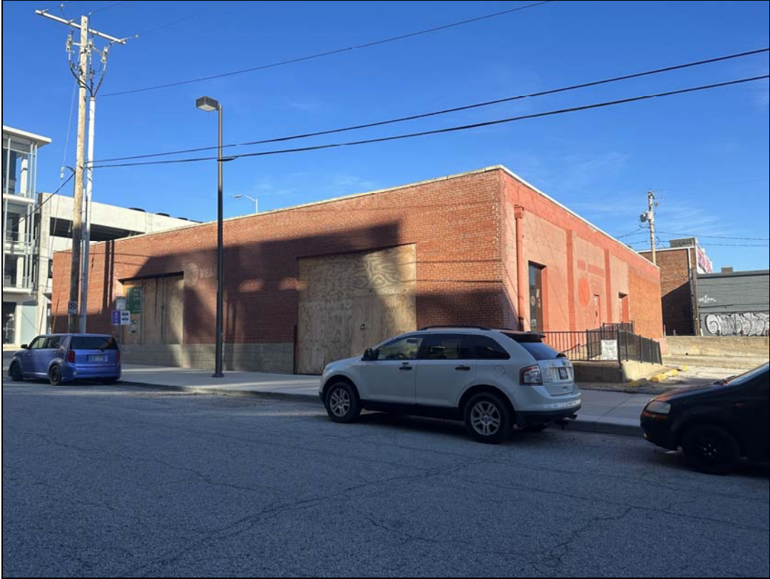
1905 Walnut Street – looking northeast at west elevation
