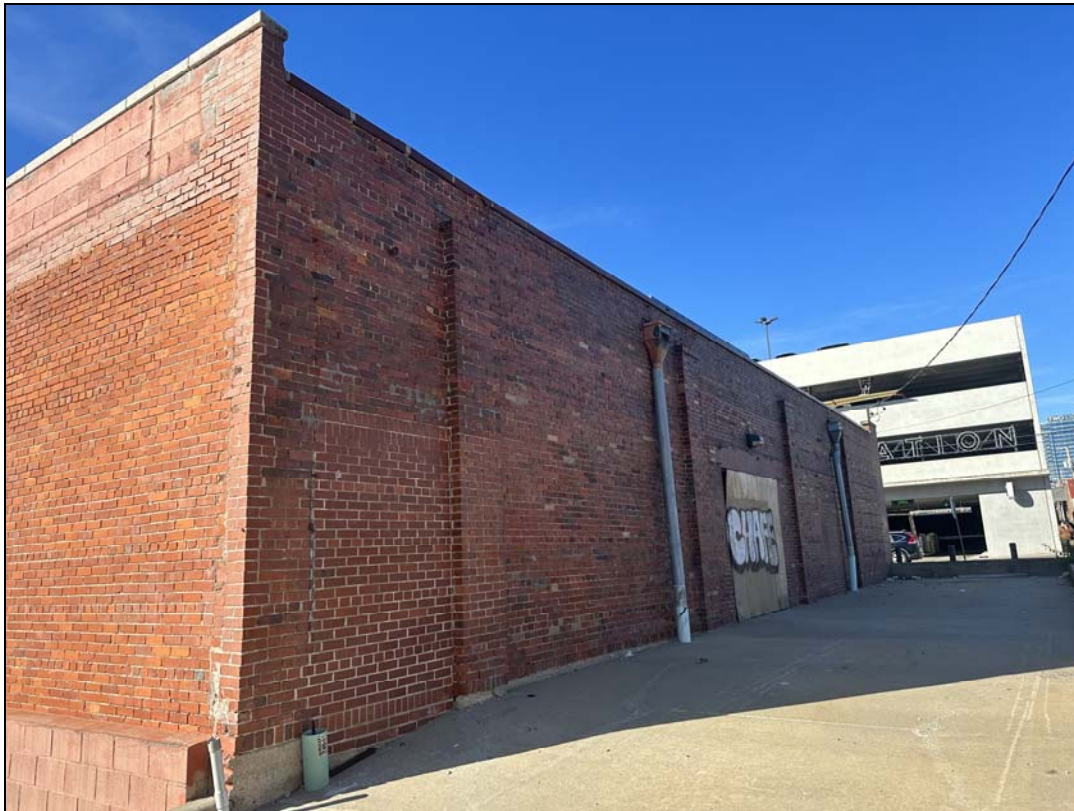
1905 Walnut Street – looking northwest at east elevation
