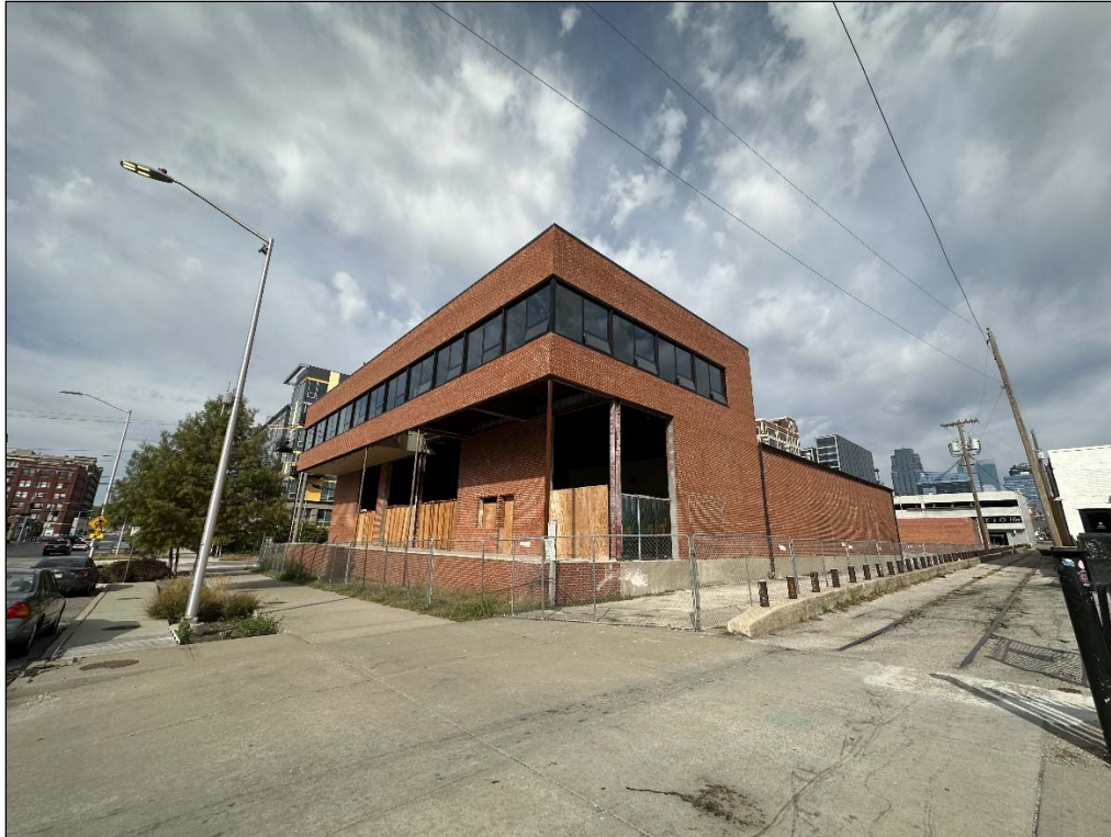
100 E. 20 th Street – looking northwest
