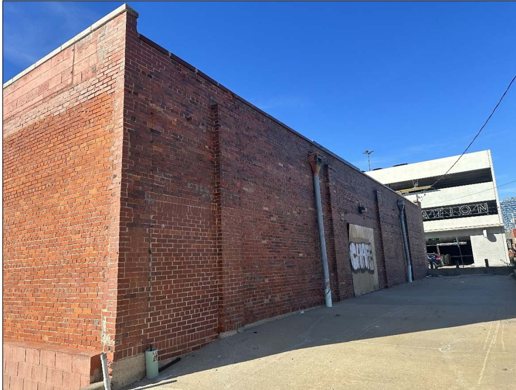
1905 Walnut Street – looking northwest at east elevation
