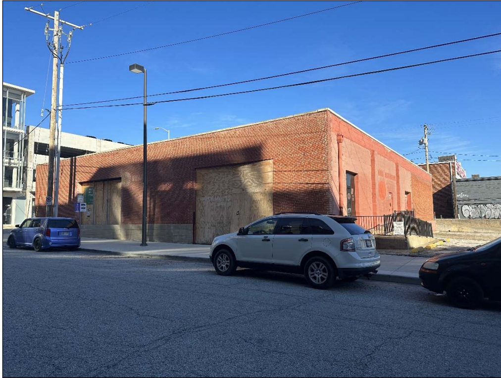
1905 Walnut Street – looking northeast at west elevation
