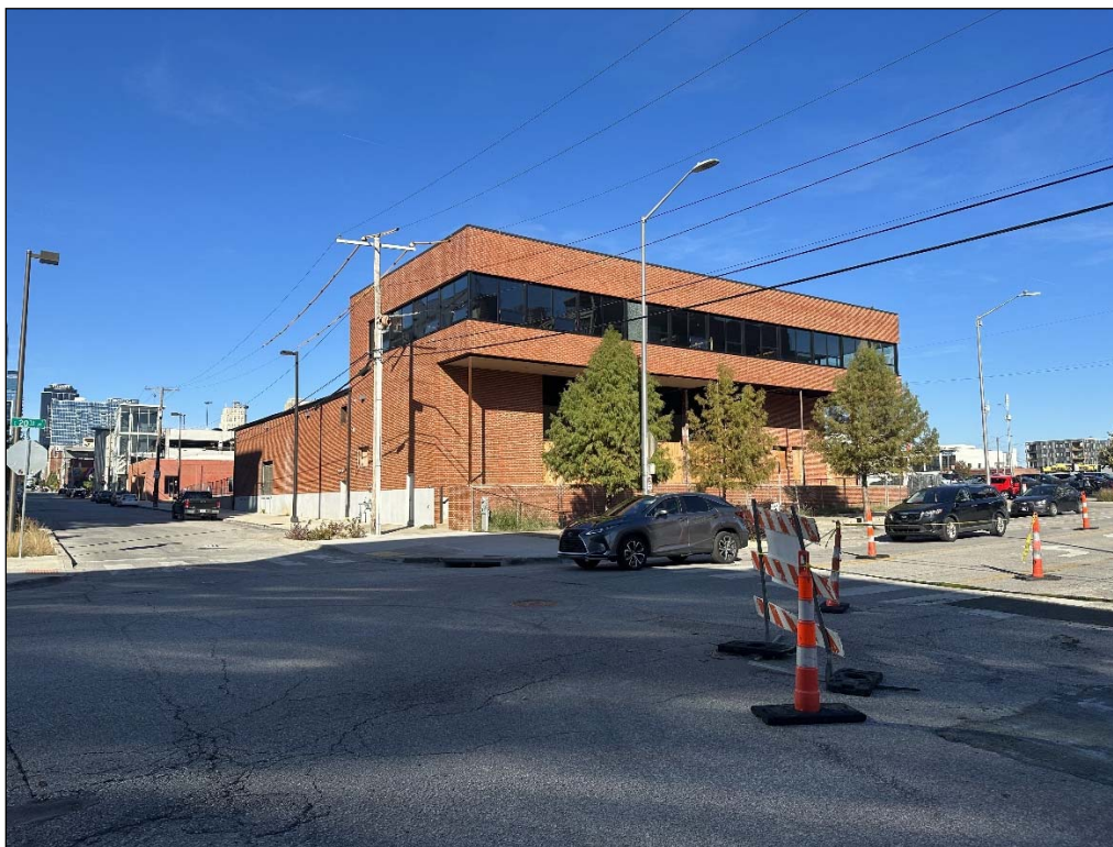
100 E. 20 th Street – looking northeast from E. 20 th Street and Walnut Street
