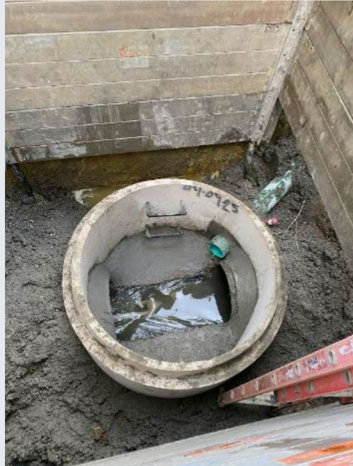
5-Foot Diameter Manhole Replacement Before and After
