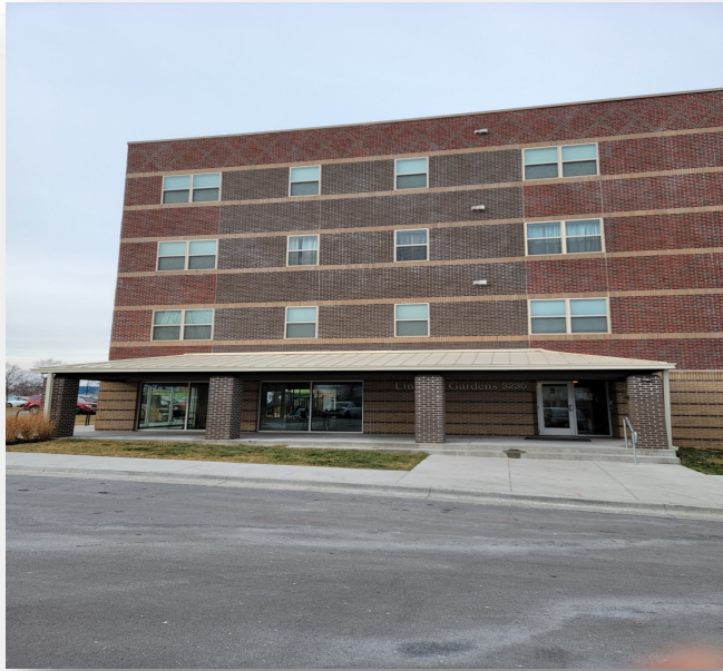
Linwood Gardens, a 32-unit property adjacent to Linwood Presbyterian Church on Linwood Boulevard and Michigan Ave
