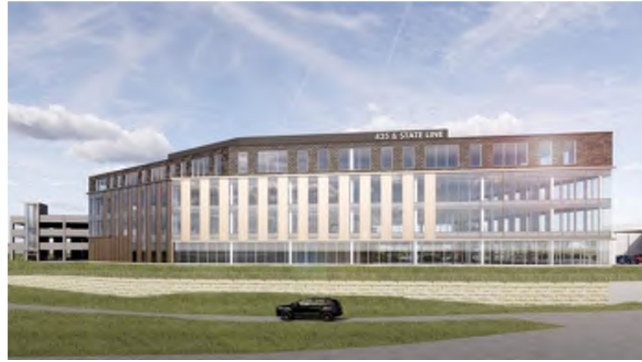
View looking East
