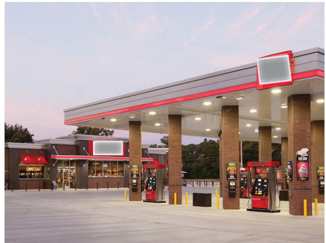
Example of C-Store Canopy
