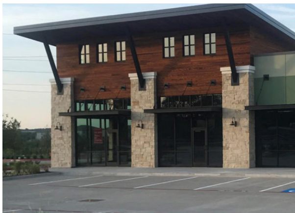
Example of Sloped Roof with Muted Tones
