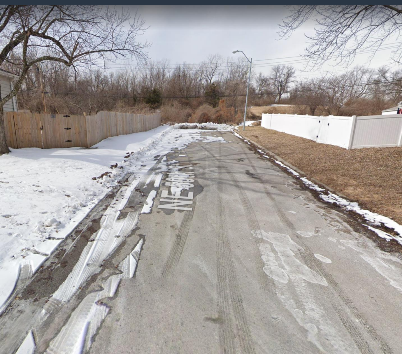
View looking west on NE 50 th St (to be vacated)
