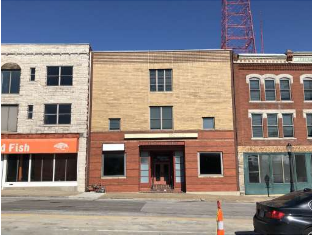
Atrium Connector West Façade (Built 1990)
