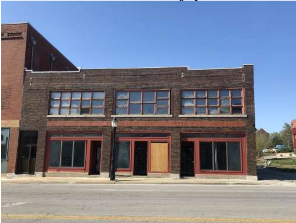
6-10 E 31 st St South Façade
