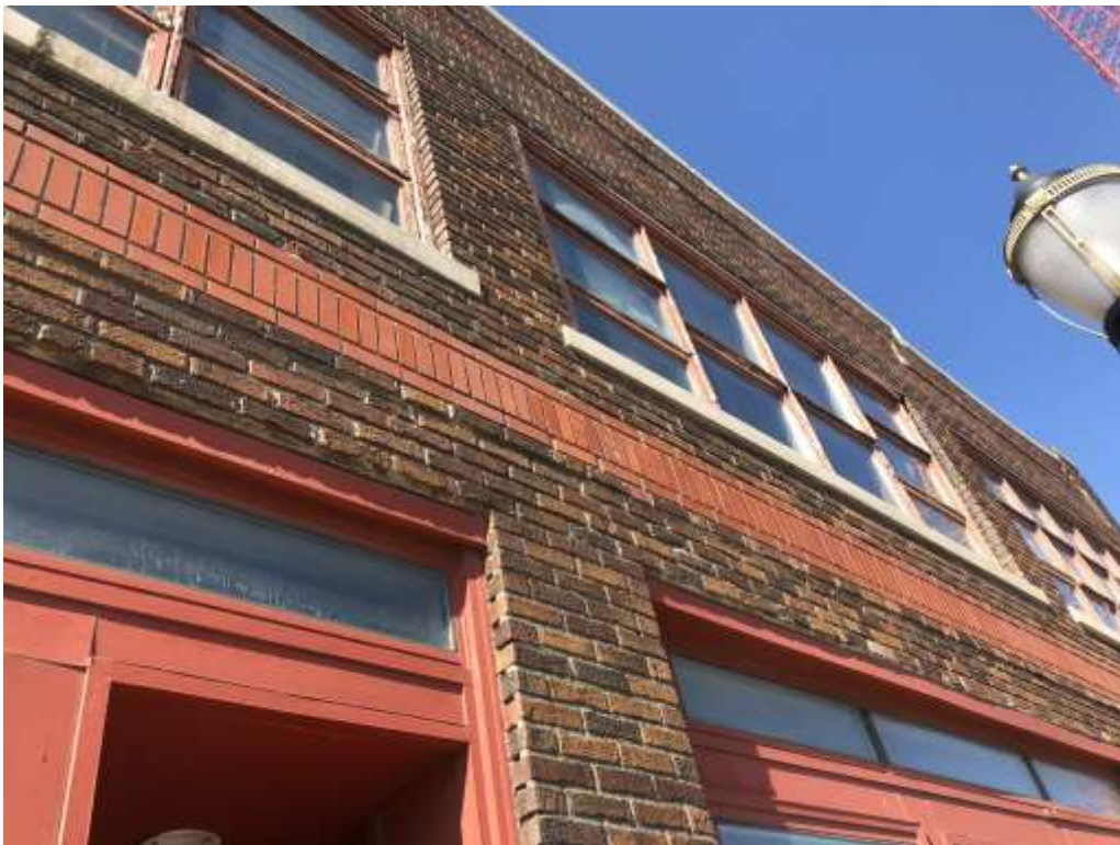
6-10 E 31 st St South Façade Detail
