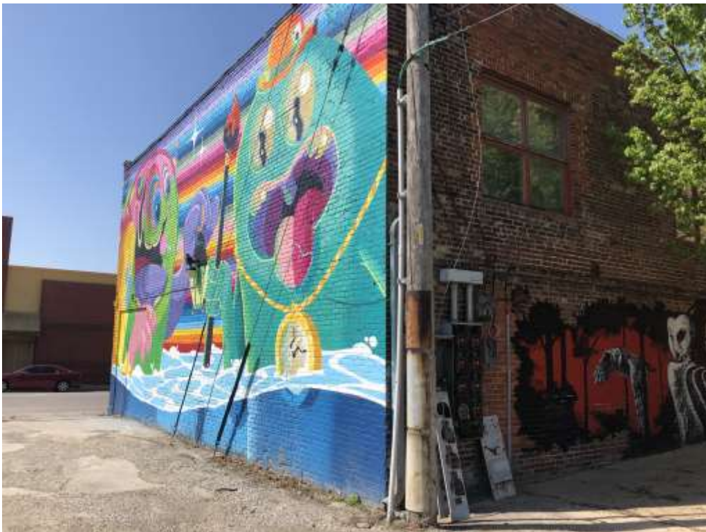
6-10 E 31 st St East Façade
