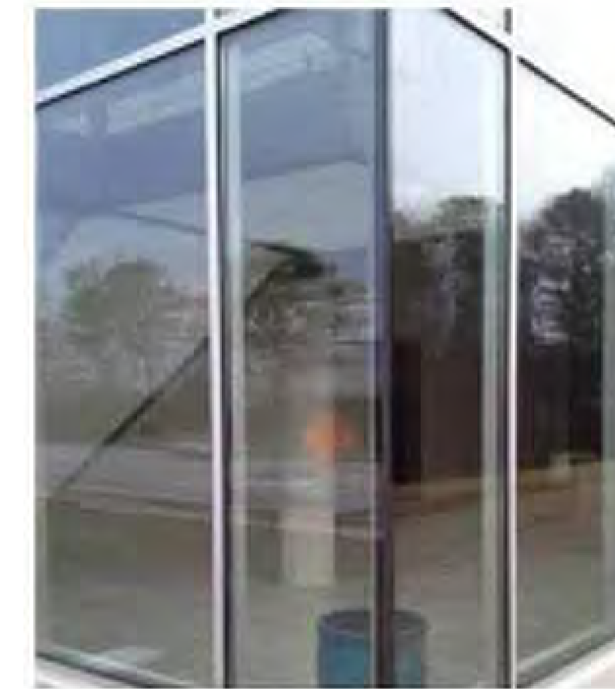
CURTAINWALL / STOREFRONT SYSTEM
