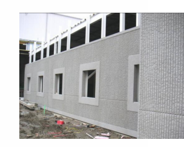
PRECAST FORMLINER PANEL
