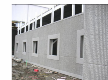
PRECAST FORMLINER PANEL
