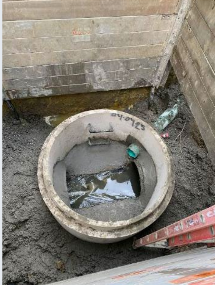
5-Foot Diameter Manhole Replacement Before and After
