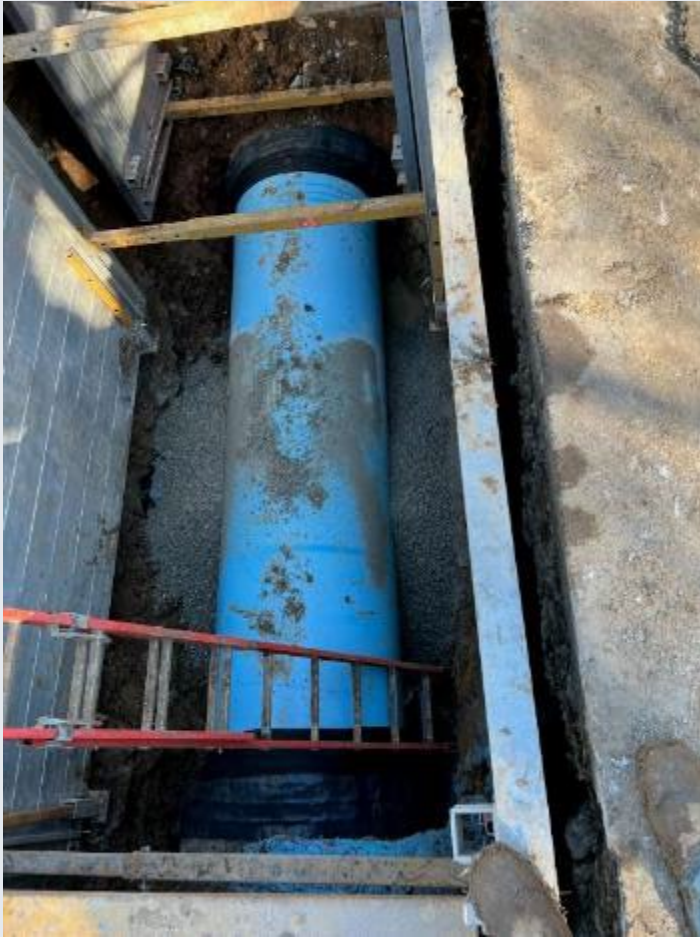
42-Inch Sewer Replacement
