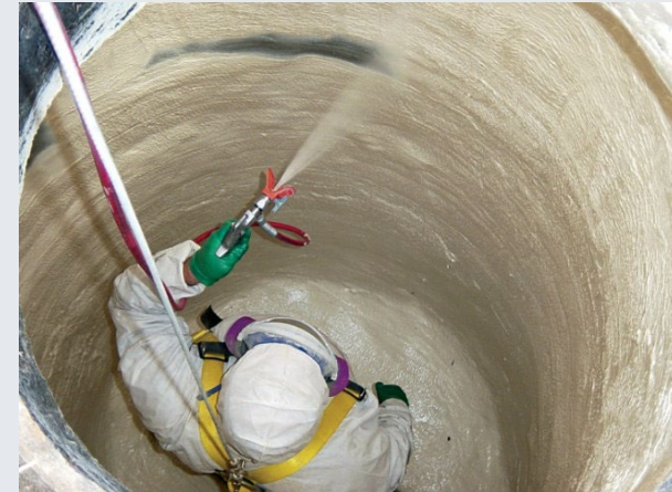
Manhole Rehabilitation
