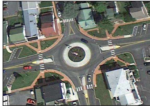
(Source: PennDOT Local Technical Assistance Program)
