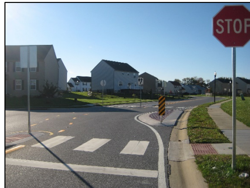
(Source: Delaware DOT)
