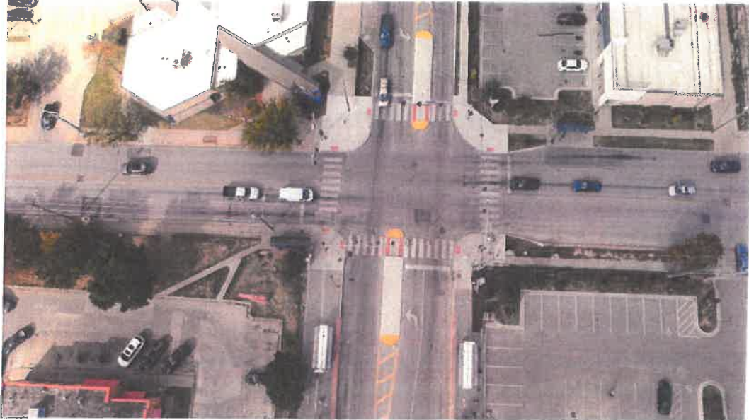
Figure 1 – Kansas City Vision Zero intersection improvements at Prospect Avenue and 31st Street. Improvements included high visibility crosswalks, pedestrian refuge islands and curb bump outs.
