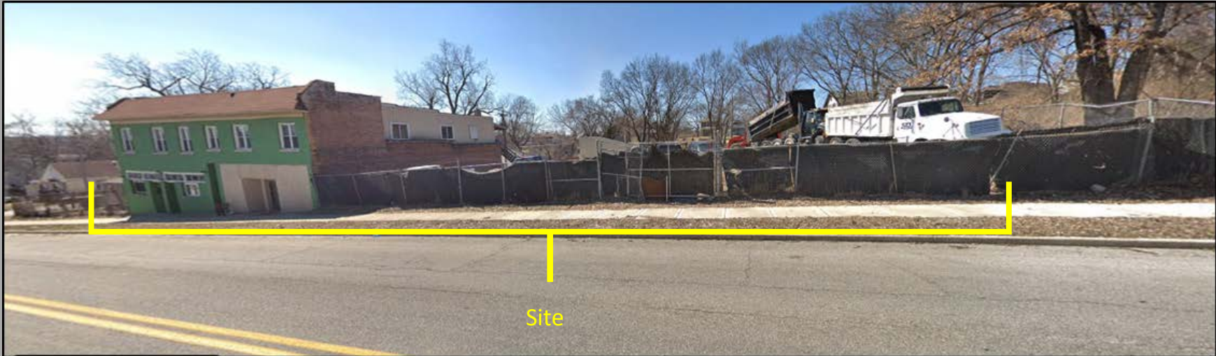
Existing street view
