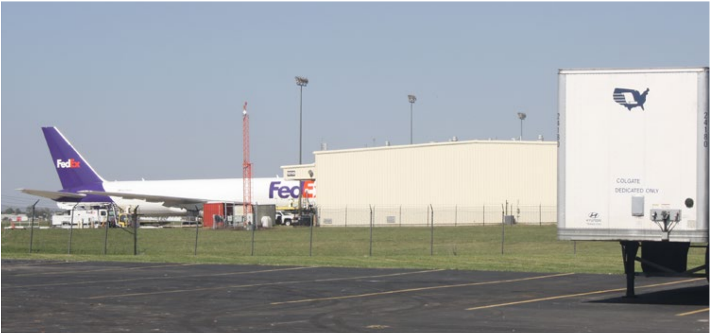
FedEx Hangar at MCI, October 2025.
