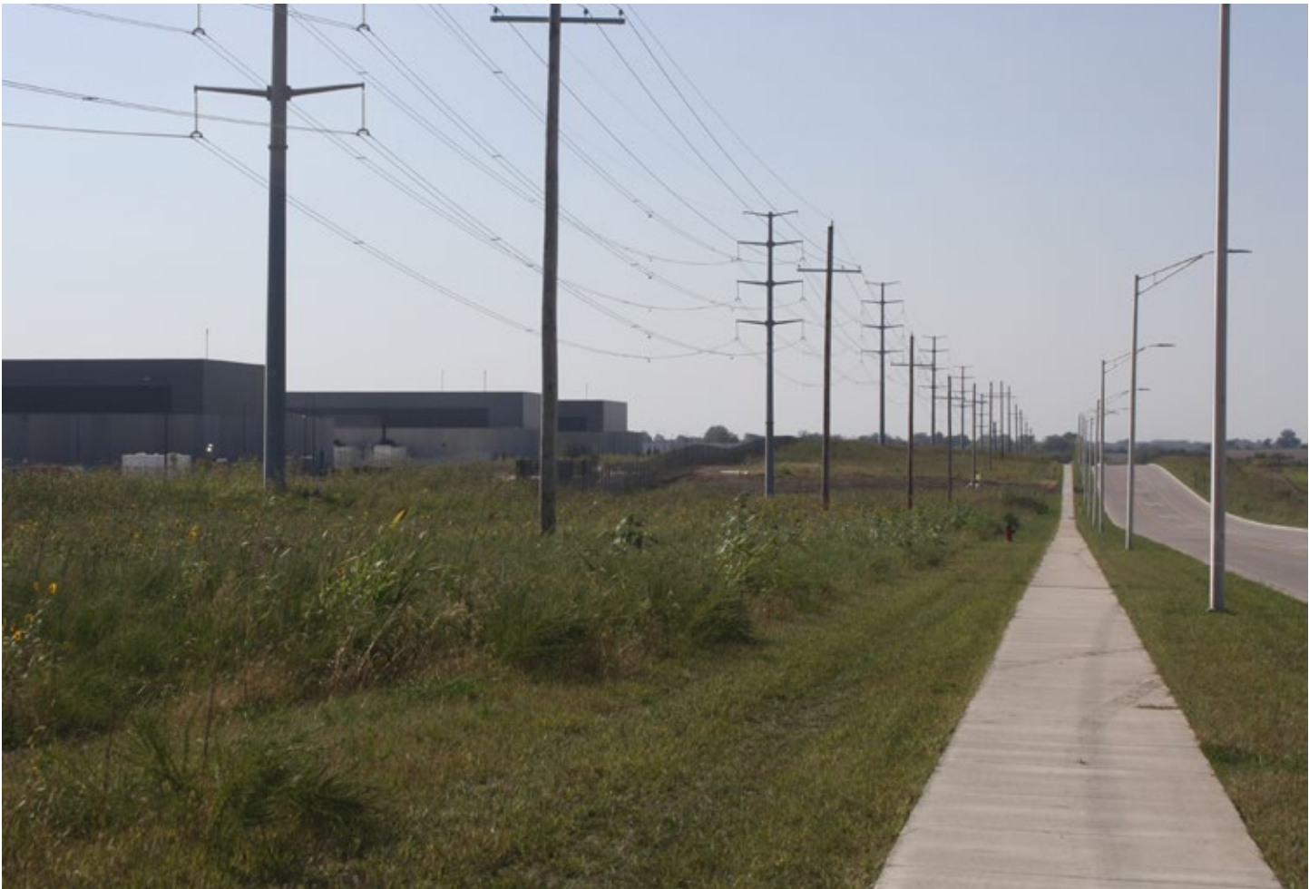
Newly constructed sidewalk in KCI Area, October 2025.
