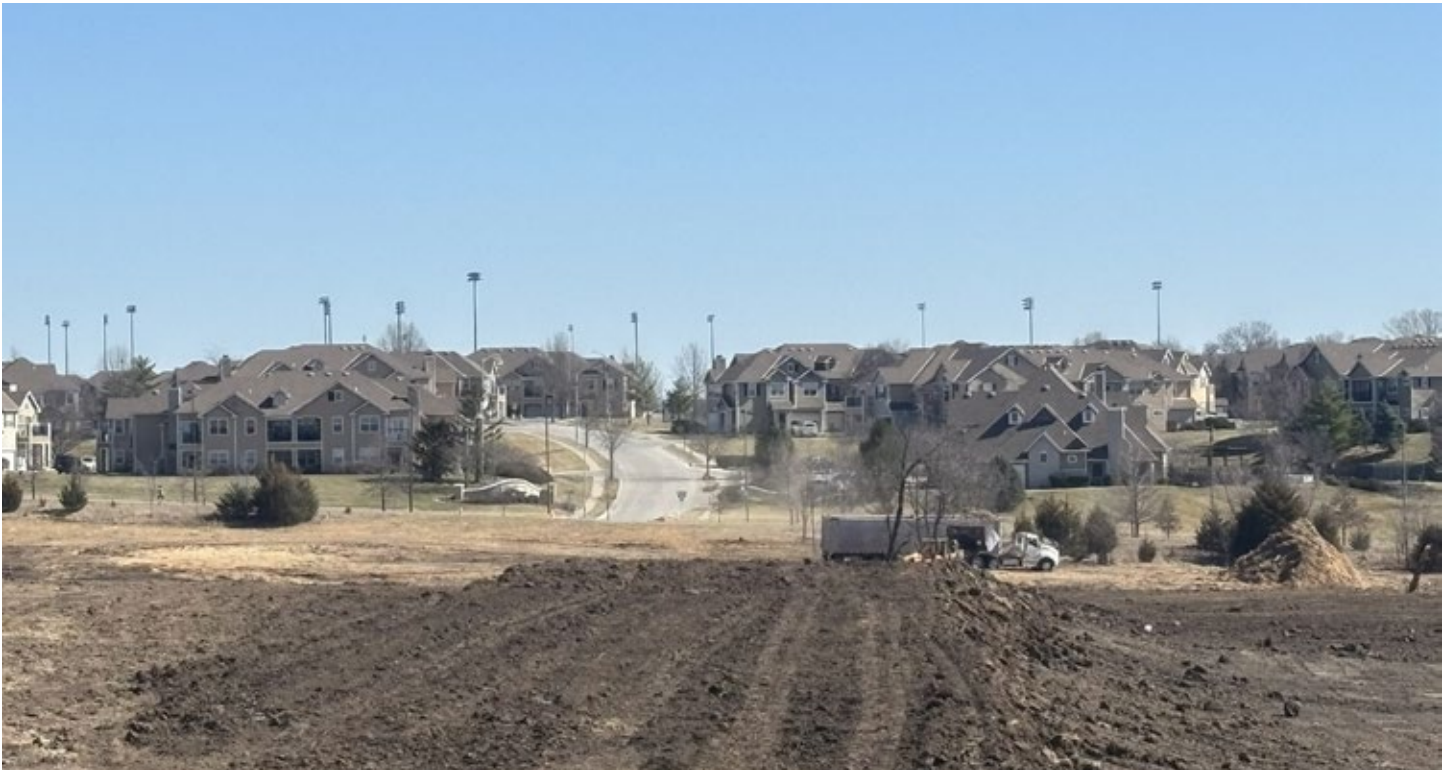
A new residential subdivision under construction, January 2026.
