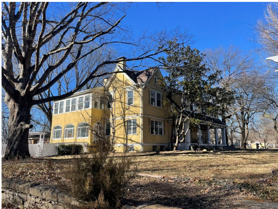
Resource No. 1: Main House (South Façade)
