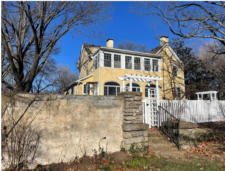
Resource No. 1: Main House (South Façade)
