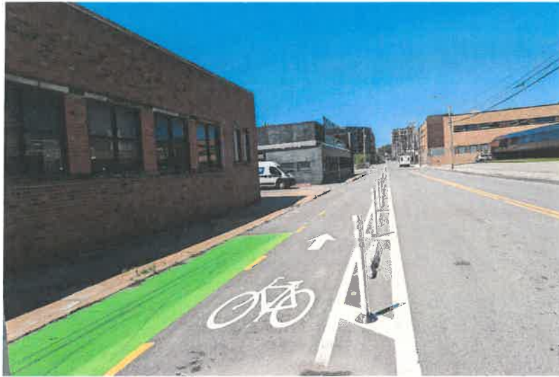
Figure 3 – Two-way cycle track using quick-build materials
